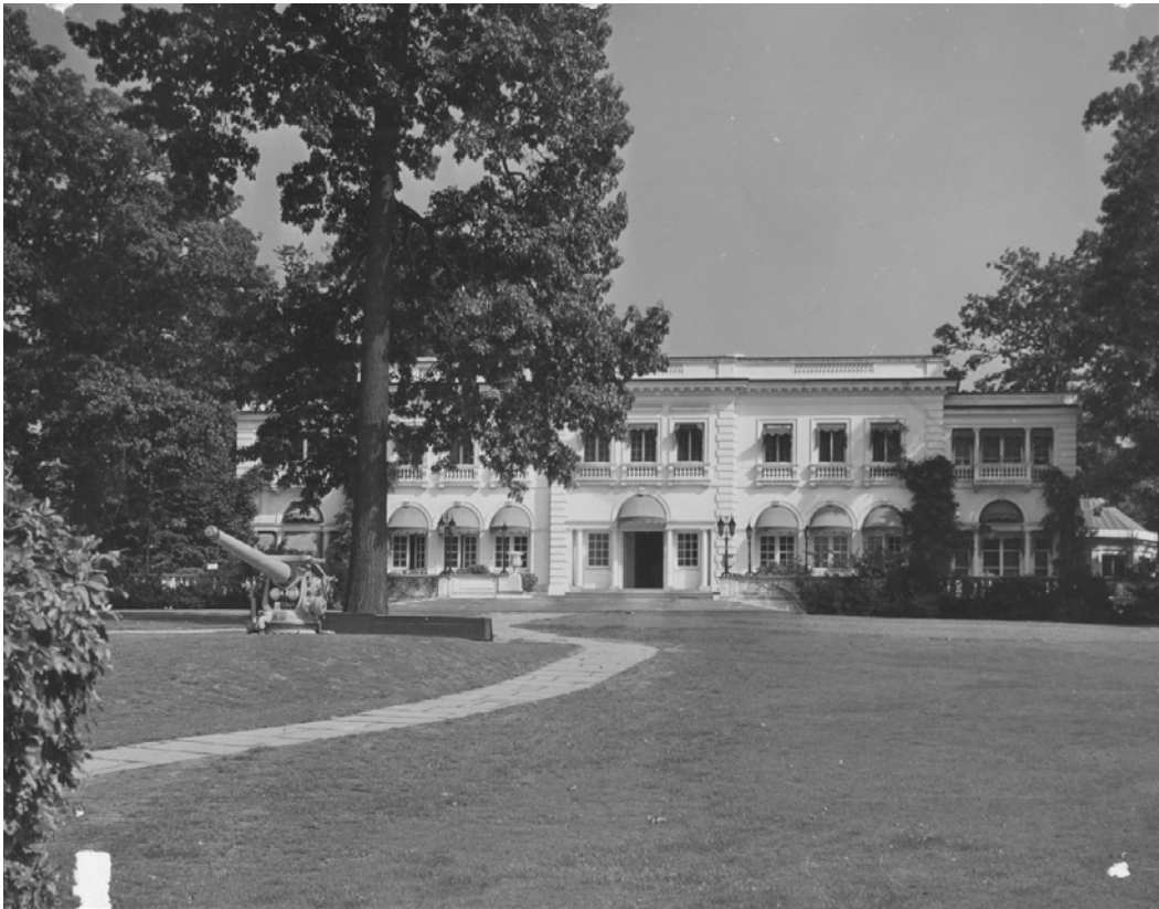
Figure B11. New flagstone walkway from Wiley Hall to pool, 1942 (USMMA Bland Library).
