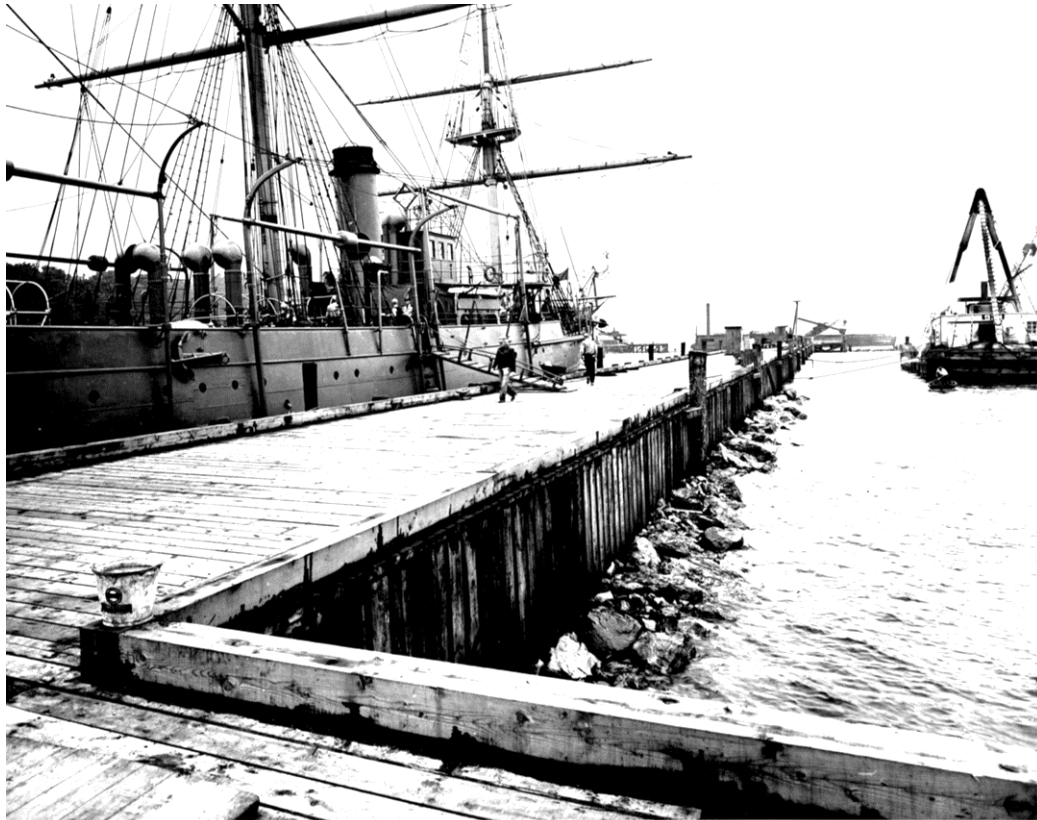
Figure B12. Completed new dock (Mallory Pier), 1942 (USMAA Bland Library).
