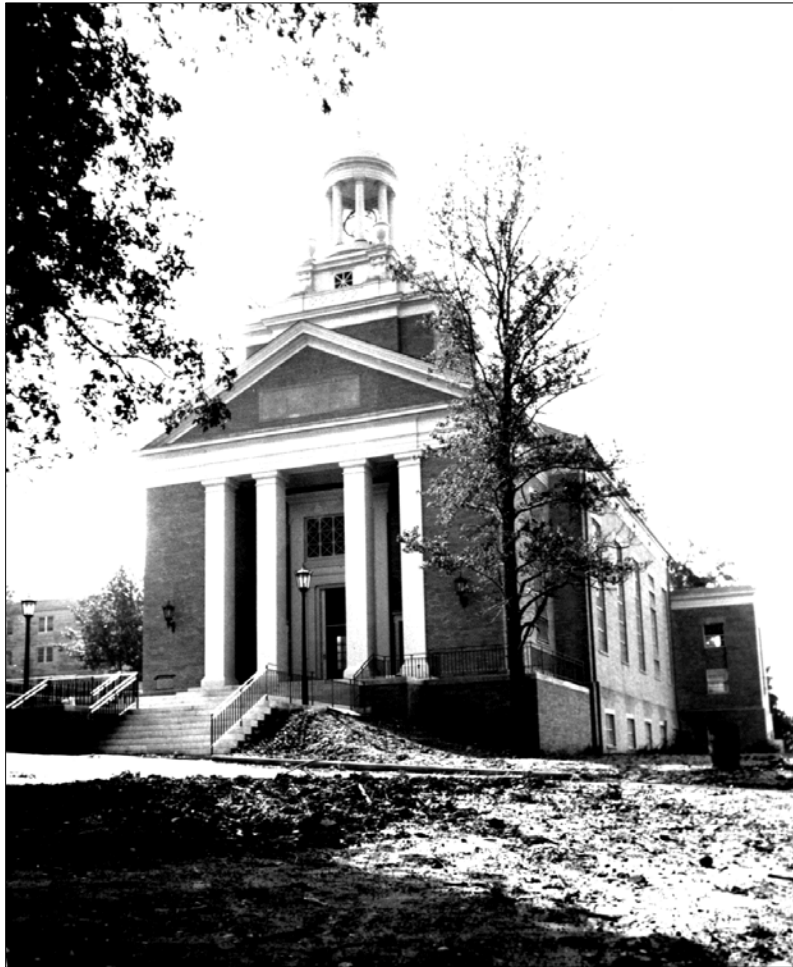
Figure B16. Chapel construction in progress, 1960 (USMMA Bland Library).
