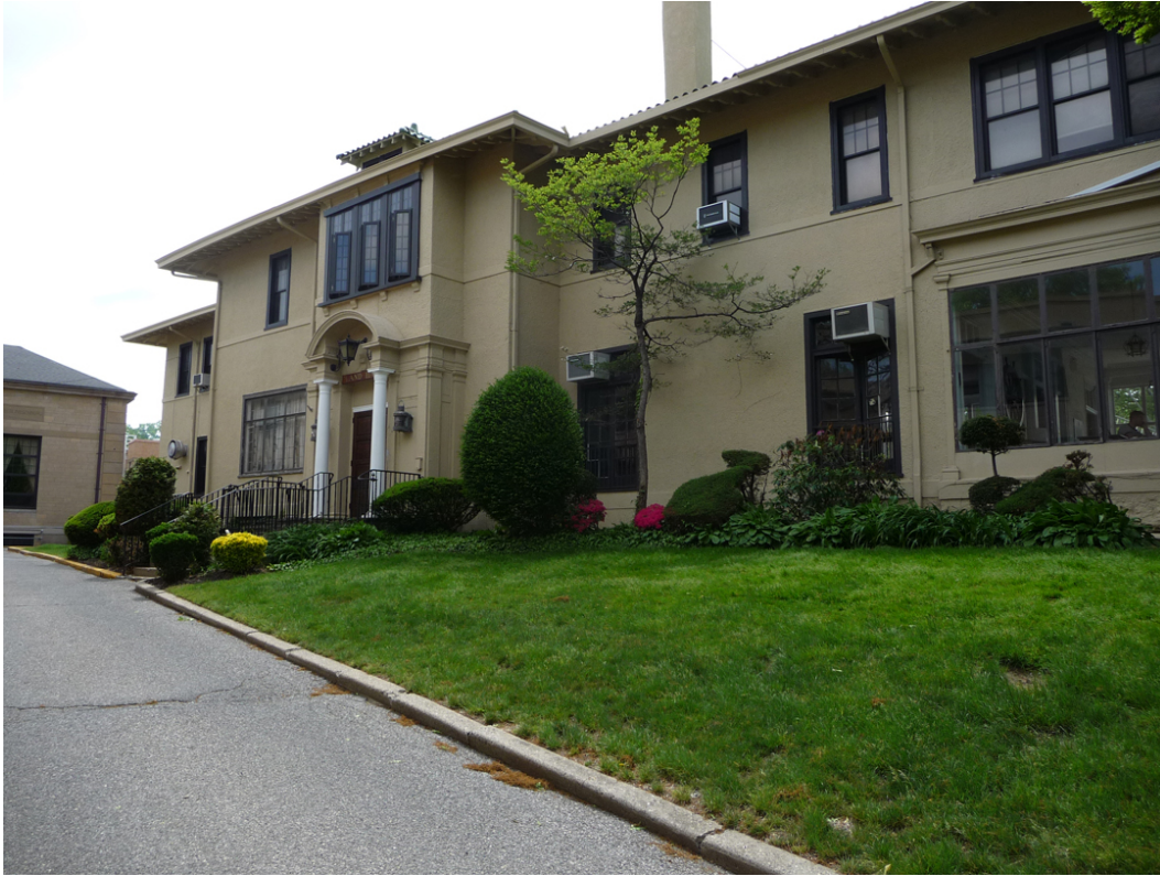
Figure 53. Schenck house (Land Hall), north facade (ERDC-CERL, 2015).
