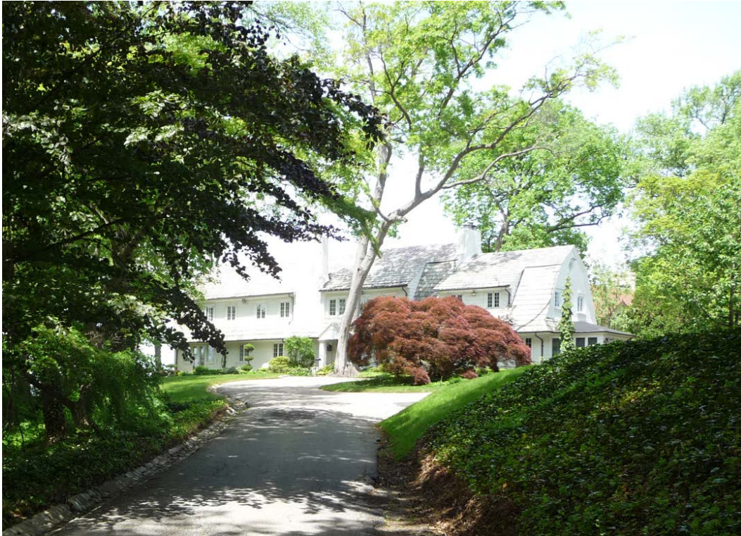
Figure 41. Entrance to Quarters A (Neiley house) (ERDC-CERL, 2015).
