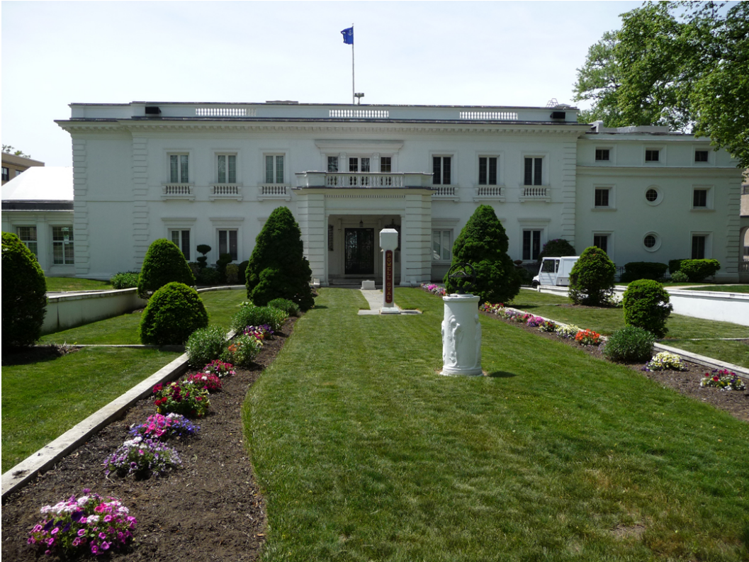
Figure 25. View of formal plantings around Wiley Hall (ERDC-CERL, 2015).
