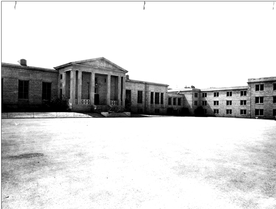
Figure B14. Newly completed parade ground (now known as Barney Square), 1943 (USMMA Bland Library).
