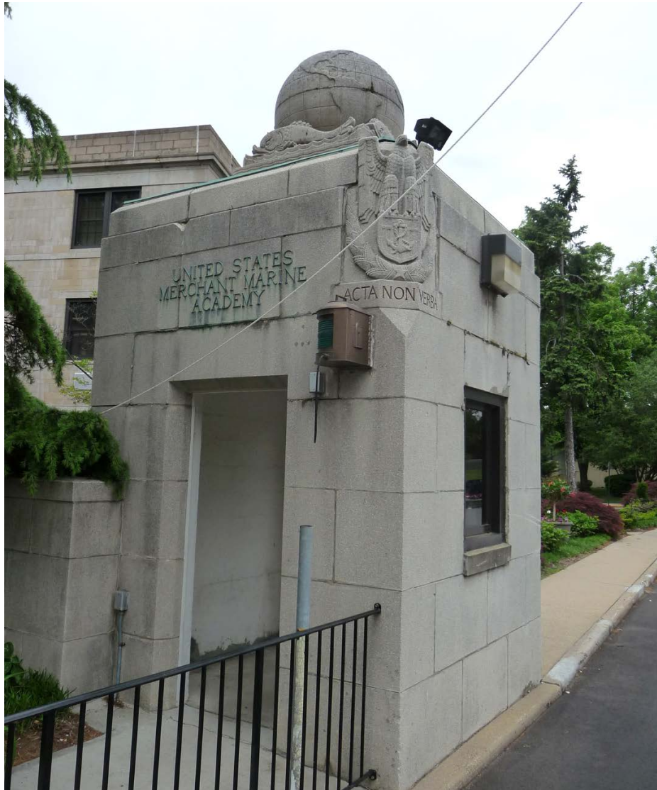
Figure 15. One of the two guard rooms forming the Vickery Gate, the main entrance to USMMA (ERDC-CERL, 2015).
