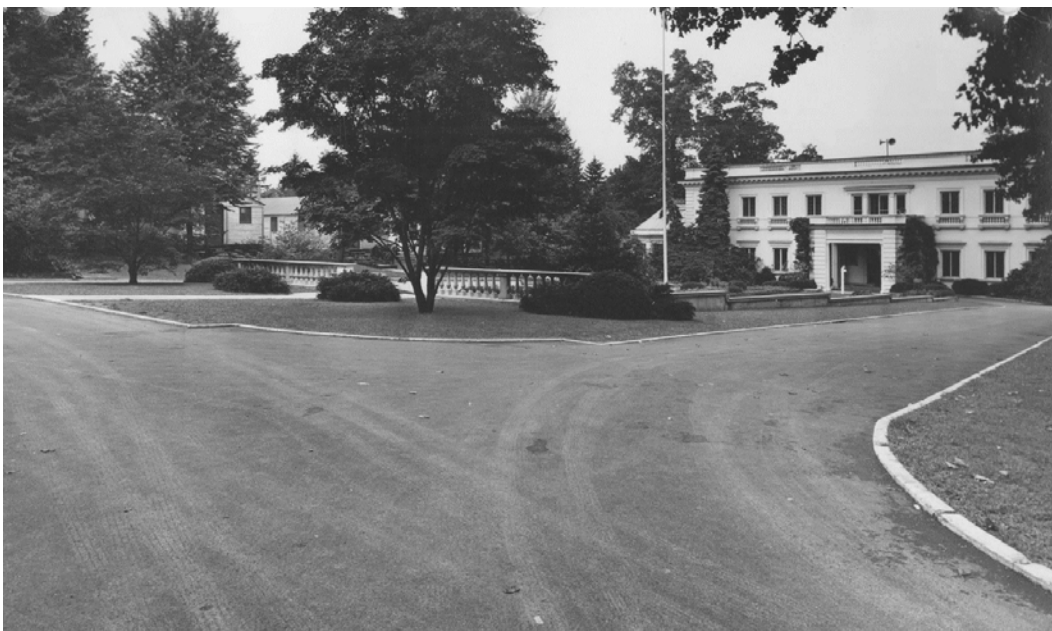
Figure 6. Newly completed asphalt drive to Wiley Hall, 1942 (USMMA Bland Library). Photo also shows existing granite stone lining the drive.
