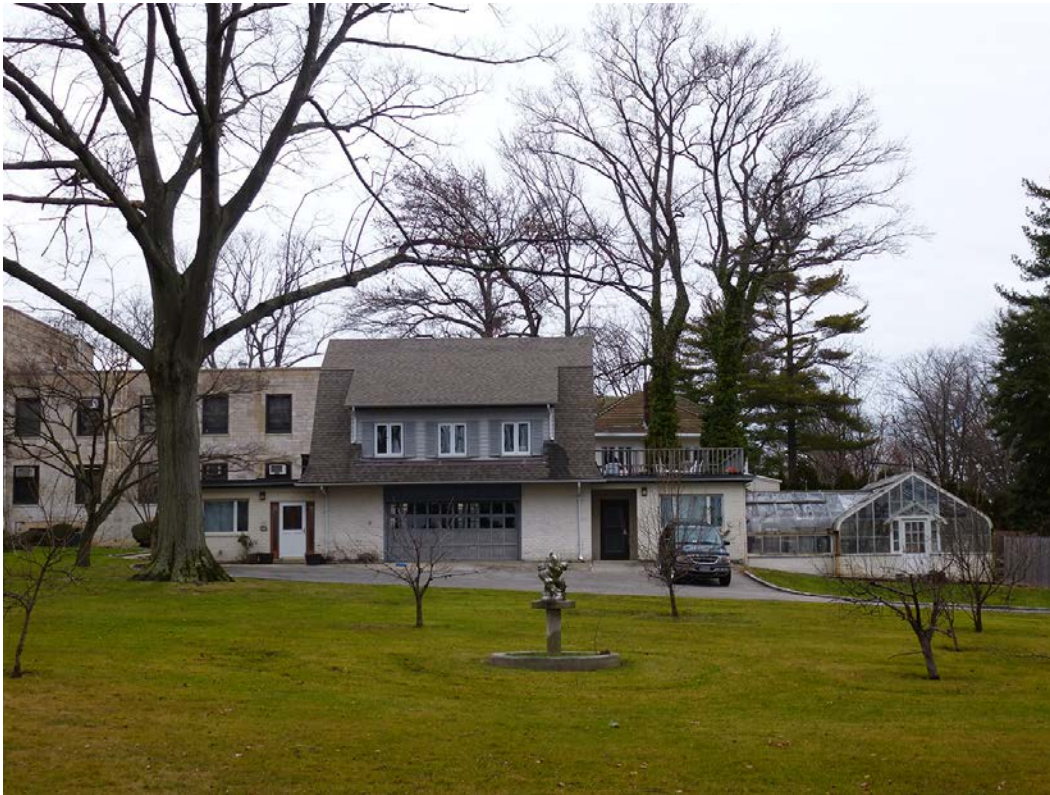
Figure 8. The Neiley house garage (Quarters J), south facade (ERDC-CERL, 2013).
