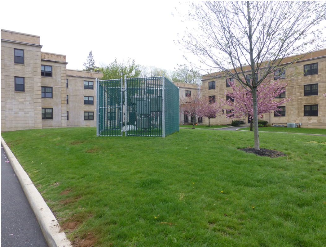
Figure 137. New chain-link style of fencing material in quad area of the USMMA Historic District (ERDC-CERL, 2017).
