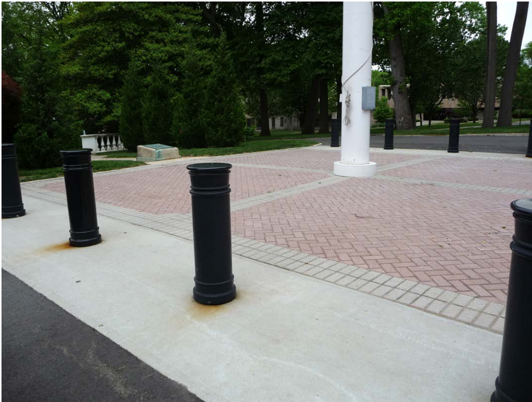
Figure 92. Bollards by flagpole (ERDC-CERL, 2015).
