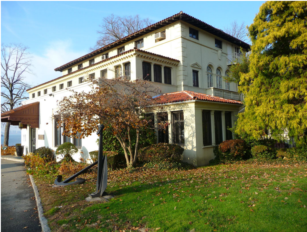
Figure 50. Vegetation around foundation of Barstow mansion (currently the American Merchant Marine Museum; ERDC-CERL, 2013).
