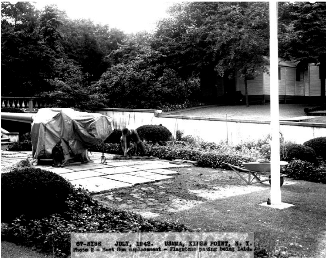
Figure 64. Training gun placement with flagstone paving being laid adjacent to flagpole, 1942 (USMMA Bland Library). Note CCC buildings in background. Flagpole was moved in 1943 to its current location.
