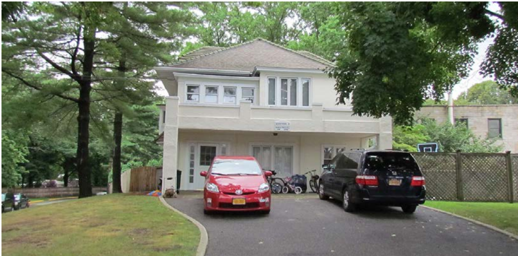
Figure 11. View to the south of Meighan house garage (Quarters K) (ERDC-CERL, 2013).
