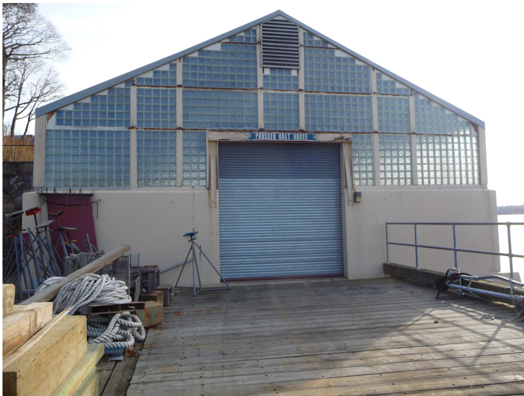
Figure 23. Marshall Pool is now Prosser Boat House (ERDC-CERL, 2013).
