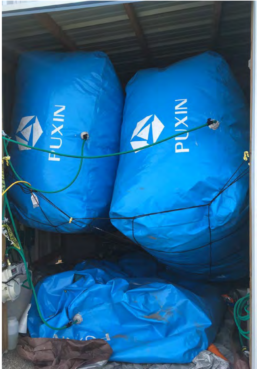
Figure 3-7 External Biogas Storage Bags
