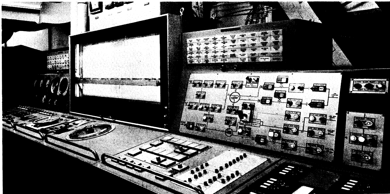
A mechanized bridge, including main engine controls (top), and a mechanized engineroom (bottom) designed for a one-man watch, place control of the ship at the fingertips of the officers in charge.
