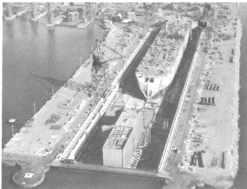
Bethlehem Steel's new 1,200-foot long shipbuilding basin at Sparrows Point, Md., can build vessels larger than 300,000 dwt.
