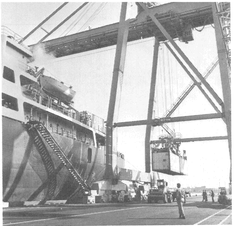
The use of containers has increased the productivity of ocean transportation systems. Containers can be lifted directly off truck chassis by cranes which deposit them on a vessel.
