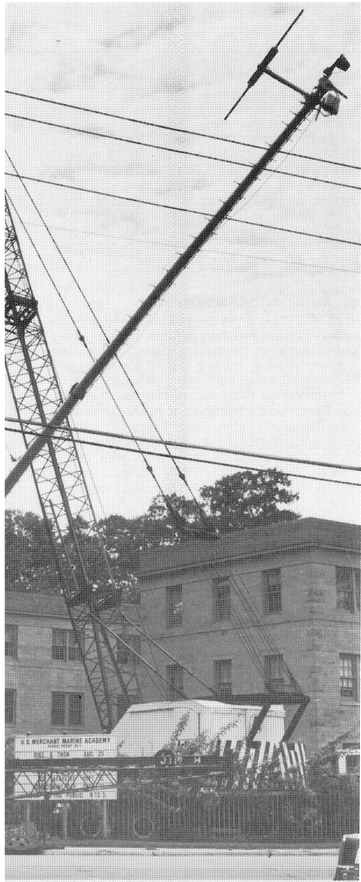
Erection of 180-foot mast with complex radar receiver mounted at top at National Maritime Research Center, Kings Point, N.Y. Radar unit monitors shipping in Long Island Sound as part of collision avoidance research project
