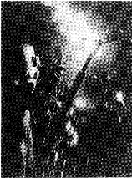
Member of workforce at Seatrain Shipyard in Brooklyn receives training in new welding techniques, one of many technological advances which have increased productivity in U.S. shipbuilding.
