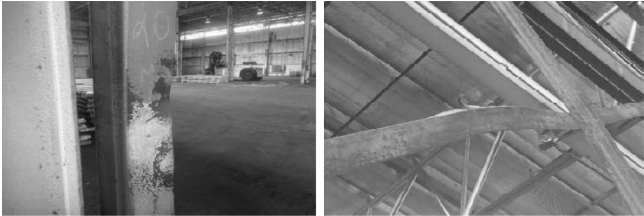
Figure 8: Impacted Column and Cross-Bracing in Warehouse A
