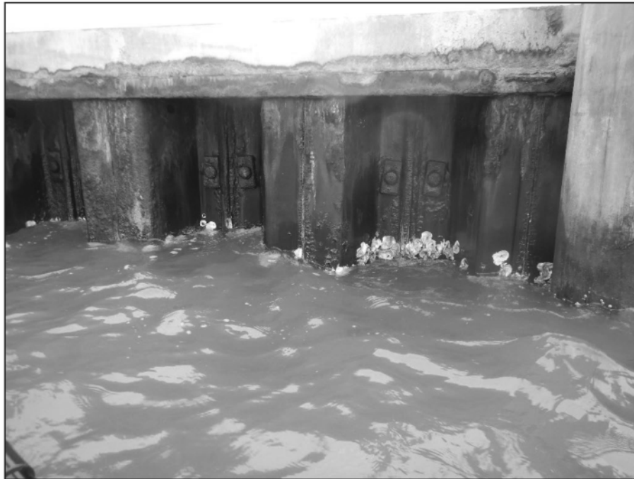
Photo 2-14 - Typical Above Water Condition of 2000s Steel (Sta 1+00 Shown)
