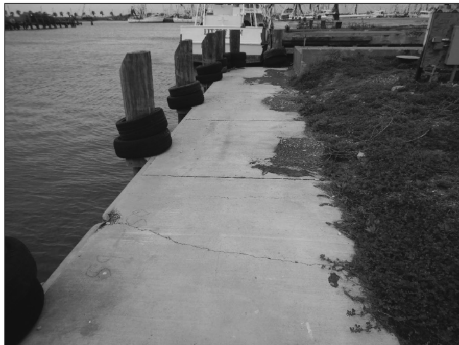
Photo 6-2 – Minor Impact Damage at Sta 59+50
