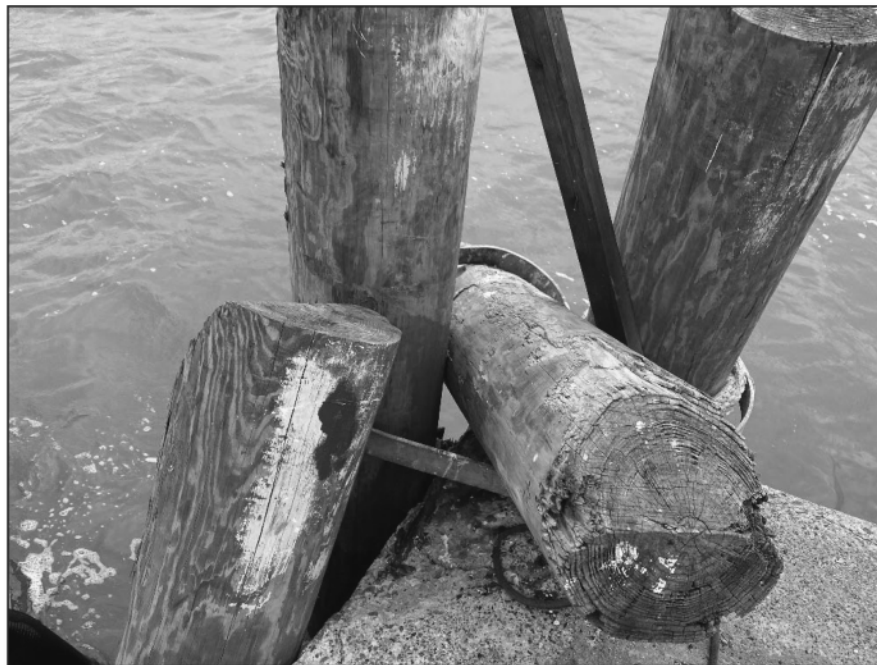
Photo 2-7 - Broken Fender Piles (Sta 31+83 Shown)
