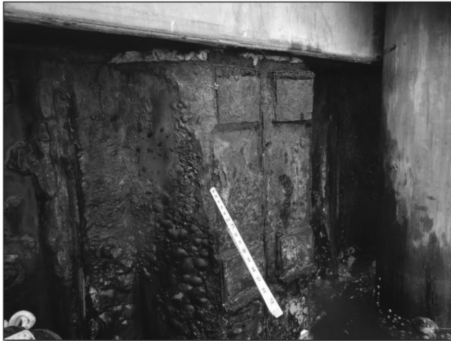
Photo 2-22 – Typical Conditions 31+90-55+91 (corrosion hole at 37+00)
