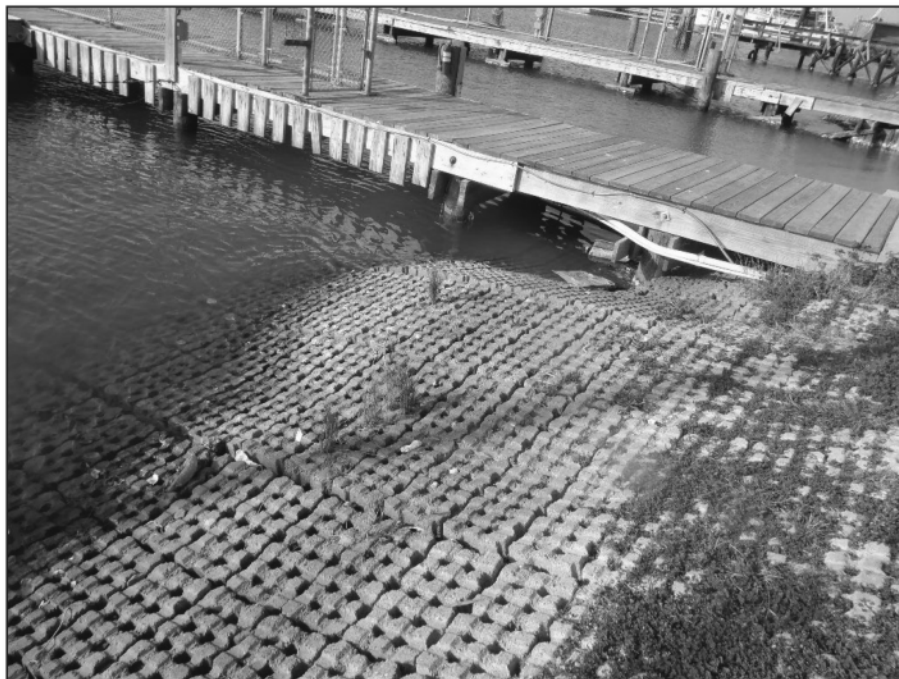
Photo 8-4 – ACM Typical Heaving
