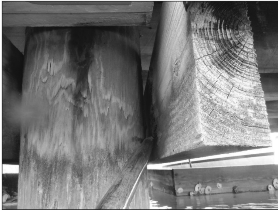
Photo 7-11 – Failed Pile Cap Hardware at Pier 4
