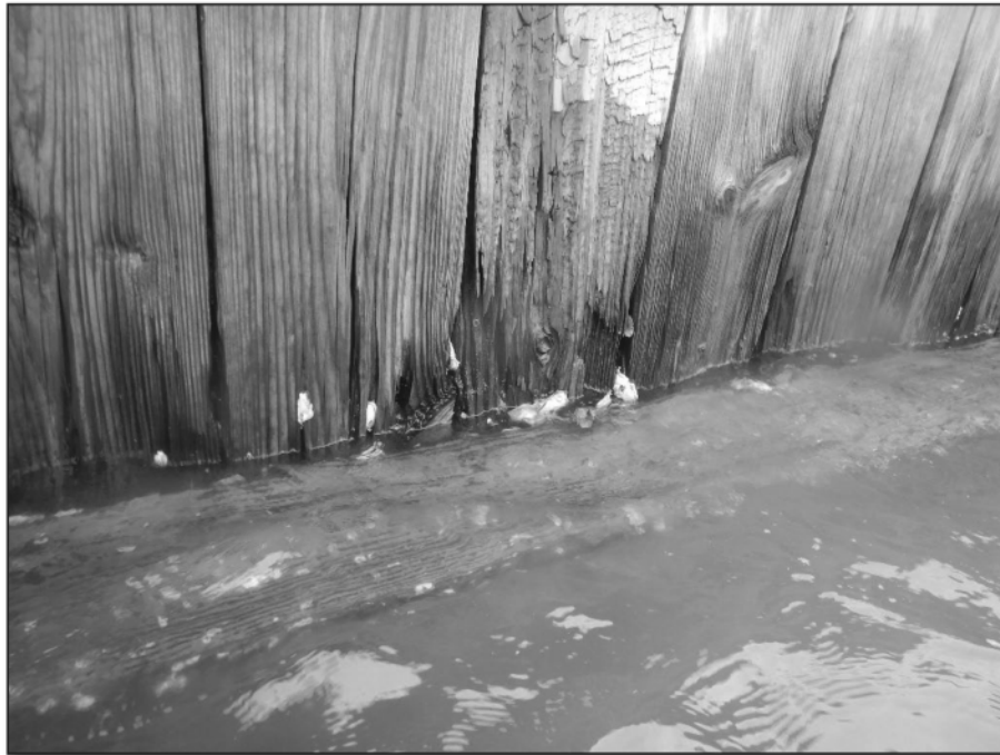
Photo 3-5 – Heavy Deterioration and Rot in Timber Sheeting (Sta 13+30-13+66)
