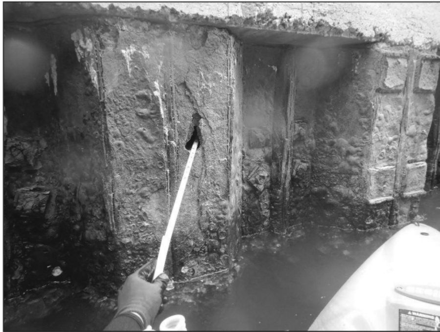
Photo 2-10 – Corrosion Holes in Sheet piling (Sta 40+00-40+50)
