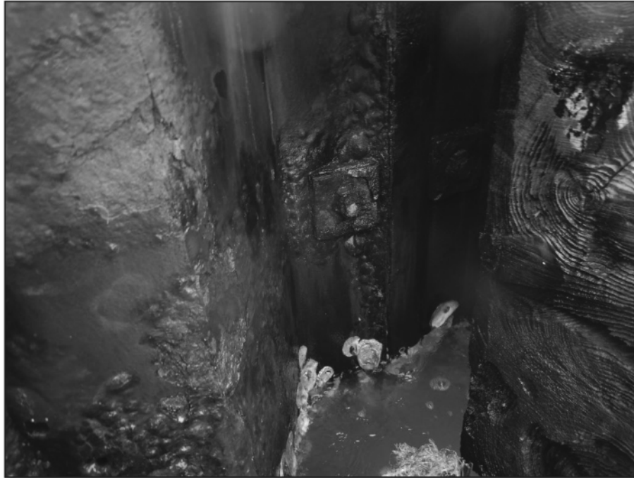
Photo 2-4 – Advanced Deterioration of Sheet Piles and Tie-Back Assembly (Sta 14+85)
