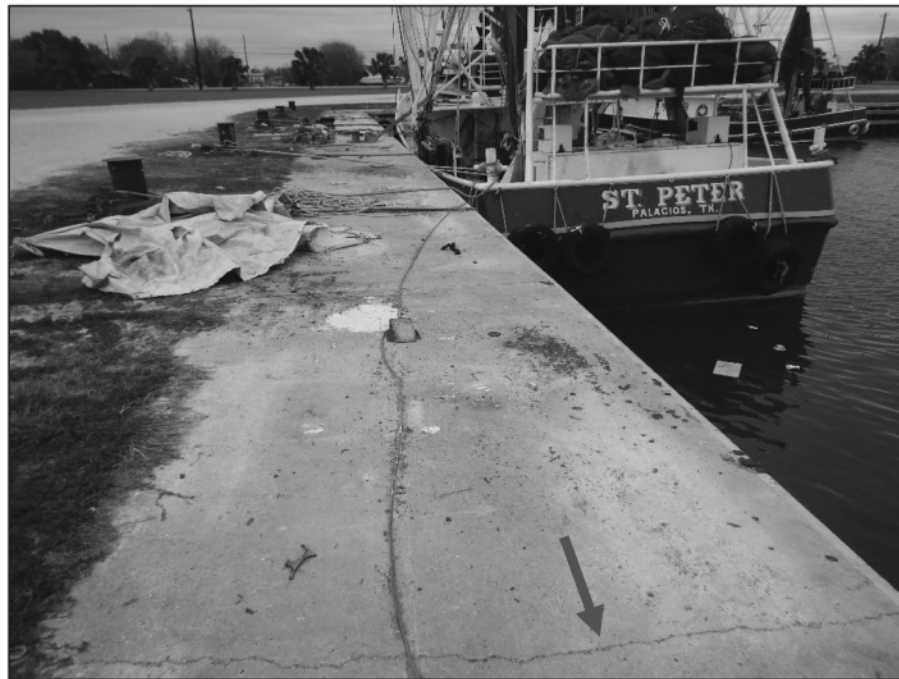
Photo 6-1 – Typical Condition of Topside, with Intermittent Transverse Cracks
