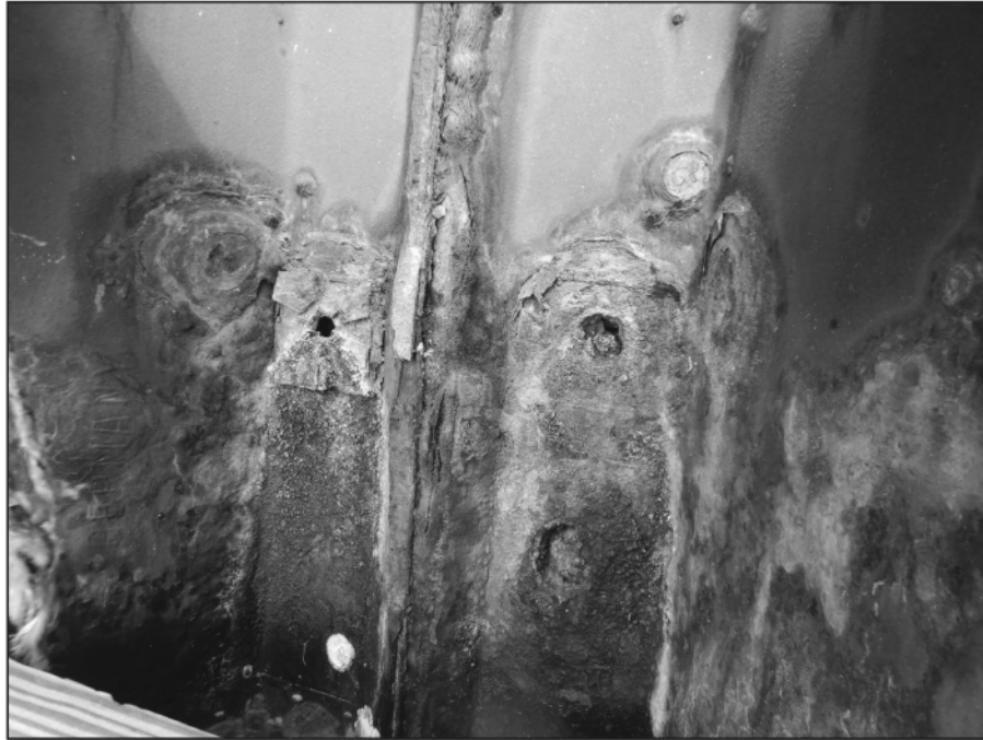
Photo 2-12 – ~100 % Loss in Tieback Assembly with Active Fill Loss (62+85-63+75)
