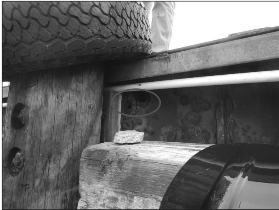
Photo 2-8 – Corrosion Holes in Sheeting at Sta 38+50
