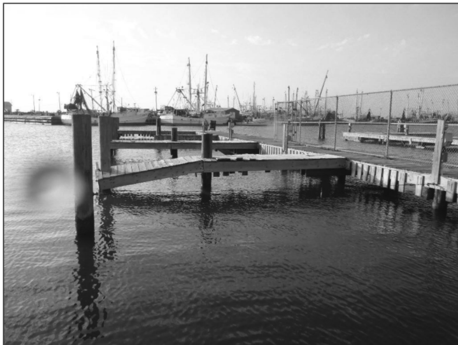
Photo 7-10 – Failed Finger at Pier 3
