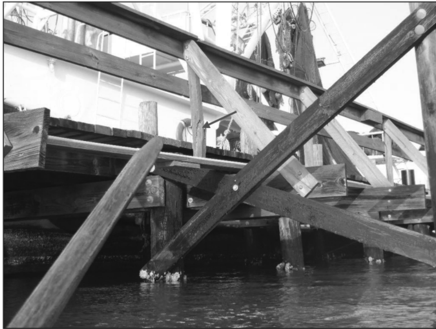
Photo 7-7 – Failed Handrail at Pier 1
