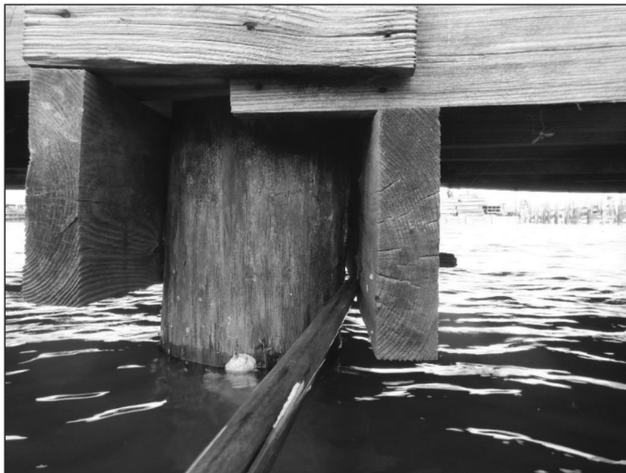
Photo 7-12 – Failed Pile Cap Hardware at Pier 5
