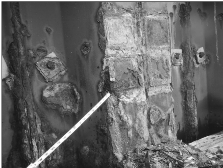
Photo 2-29 – Typical Conditions 110+80-120+50 (corrosion hole at 116+00)
