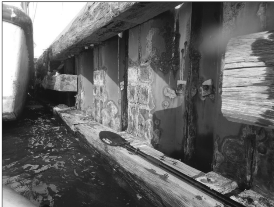
Photo 5-1 – Typical Condition of 1980s Fender System
