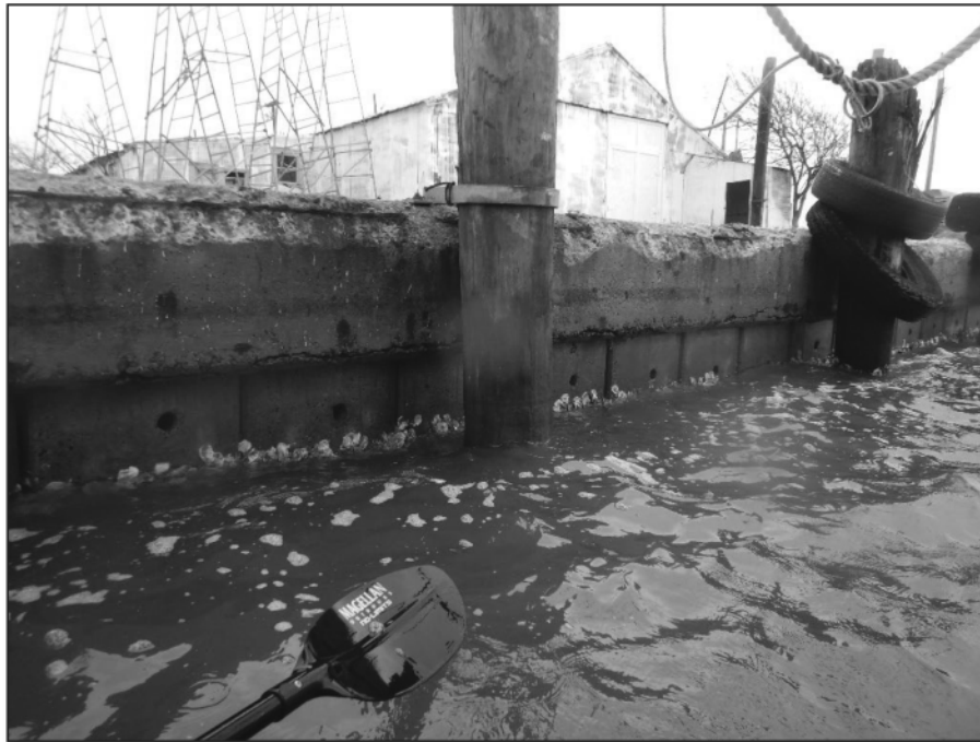
Photo 4-1 – Typical Above Water Condition of Concrete Sheet piling North of Turning Basin 1 (Sta 14+50 Shown)
