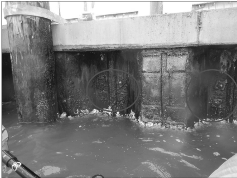
Photo 2-3 - Section Loss in Tieback Bolts and Washers between Sta 5+20-7+04
