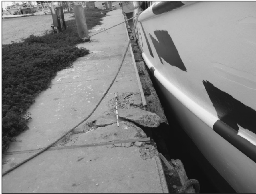
Photo 6-3 – Impact Damage at Sta 66+60
