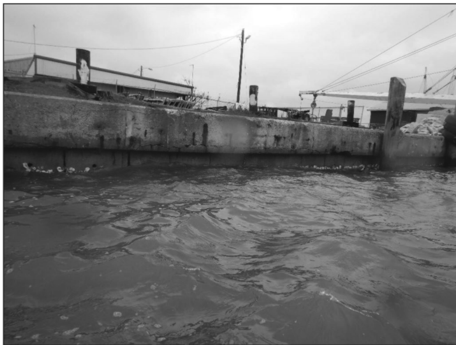
Photo 4-5 – Edge Spalls and Longitudinal Cracking with Rust Staining (Sta 28+85-31+90)
