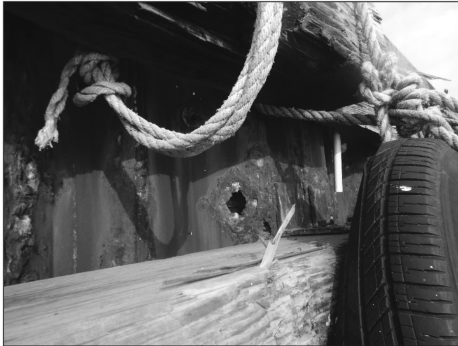
Photo 2-1 – Typical Above Water Condition of 1980s Steel with Localized Thru Hole (Sta 113+00 Shown)
