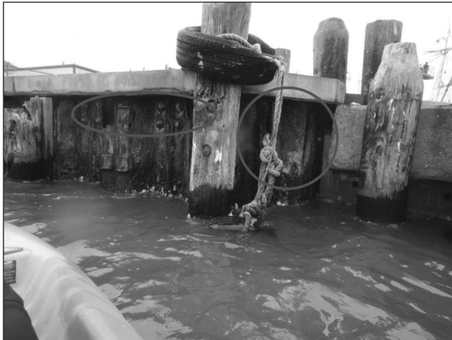
Photo 2-5 - Corrosion Holes at Transition (Sta 31+90)
