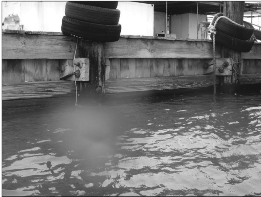
Photo 3-7 – Heavy Corrosion in Steel Fasteners at 1987 Timber Sheeting (Sta 16+60-18+48)
