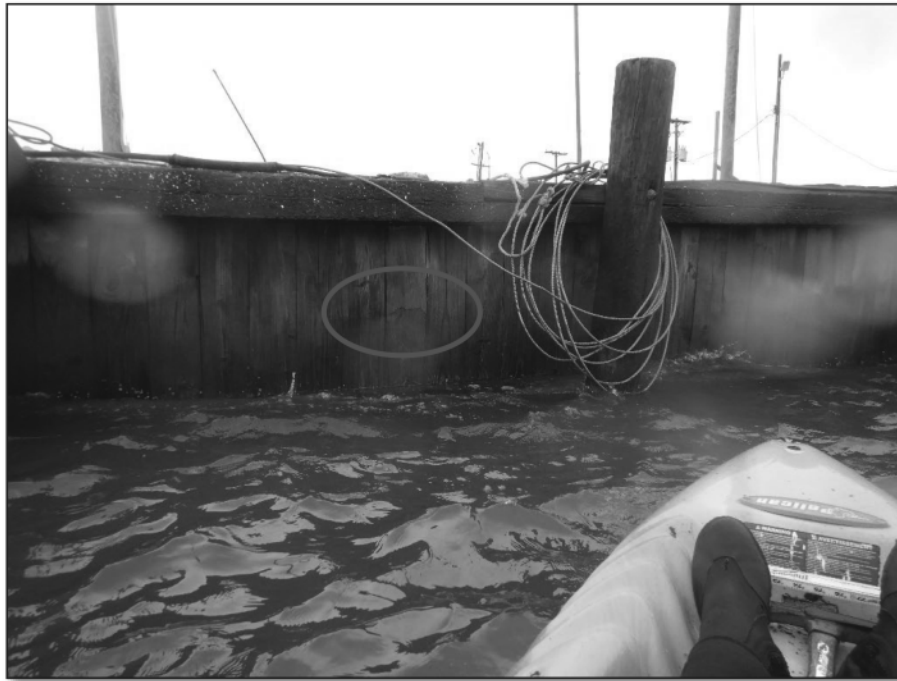
Photo 3-1 - Older Vintage Timber Sheeting Exhibiting Split Planks (Sta 12+50 Shown)
