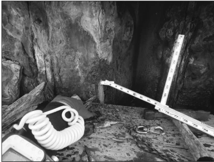
Photo 2-26 – Typical Conditions 62+85-70+00 (corrosion hole at 69+80)
