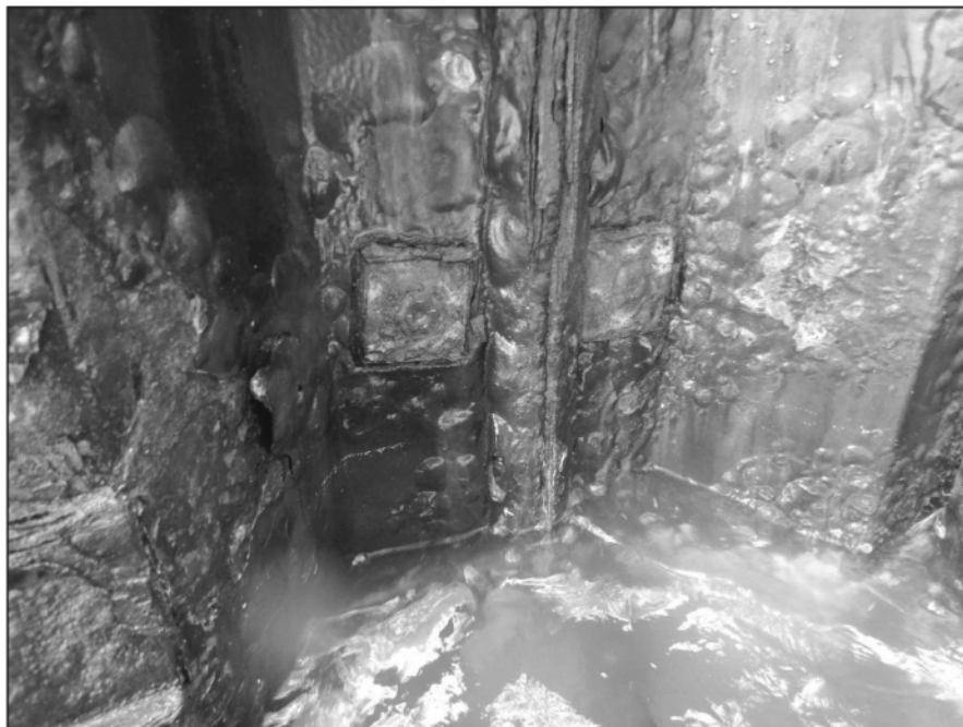
Photo 2-23 – Typical Conditions 31+90-55+91 (~100% loss of tie-back bolt heads)
