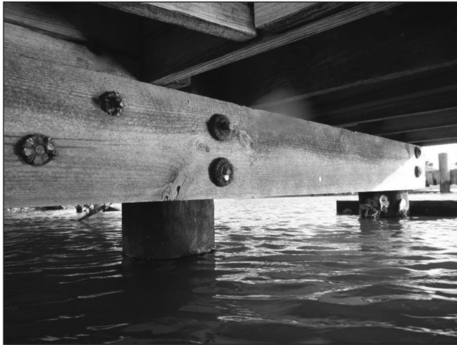
Photo 7-9 – Severe Corrosion in Pile Cap Hardware at Piers 2 and 3
