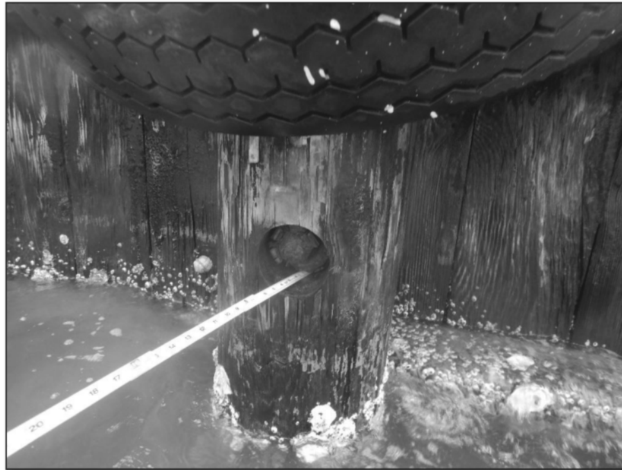
Photo 3-9 – ~100% Section Loss of the Tie-Back Rod Nuts (3+34 to 5+20)
