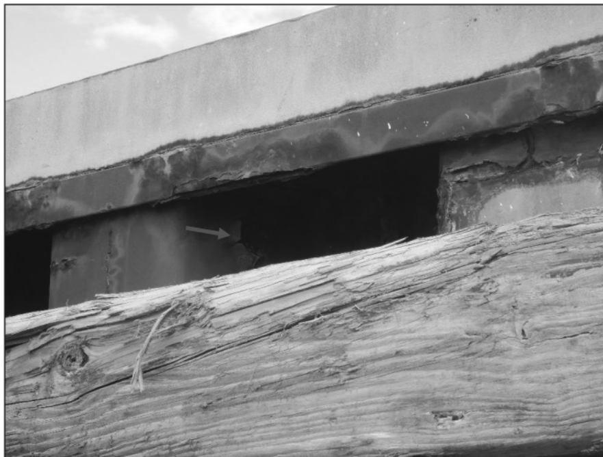
Photo 2-17 – Missing Backing Material to Lifting Holes (70+00-97+50)
