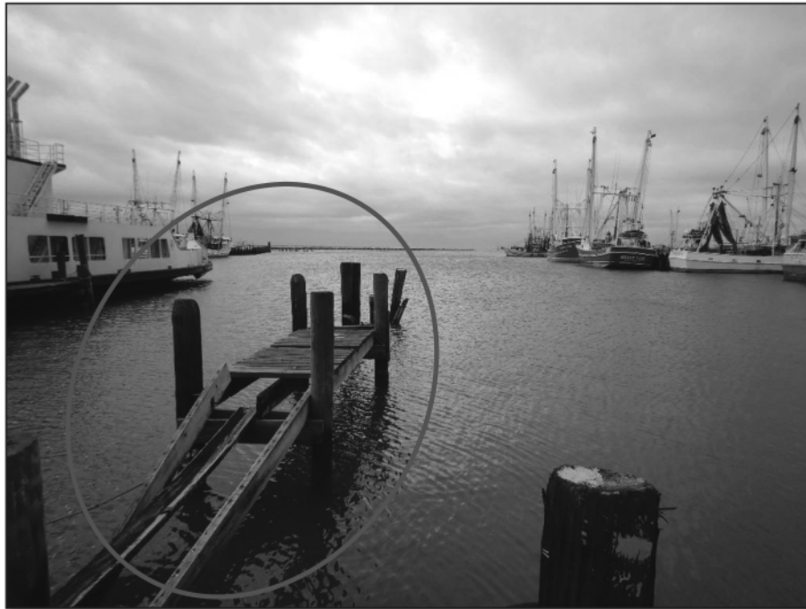
Photo 7-14 – Western Pier in State of Disrepair Adjacent to Marine Railways
