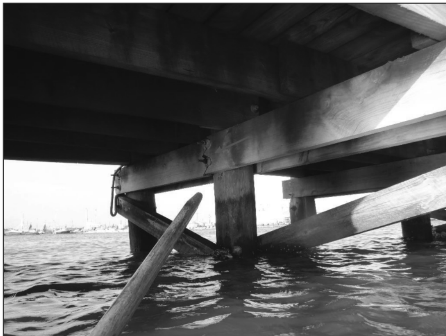
Photo 7-8 – Split Pile Cap at Pier 1
