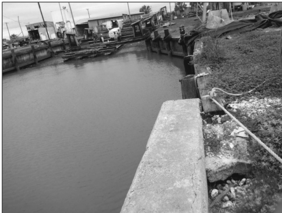
Photo 3-4 – Seaward Settlement and Sinkholes Throughout (Sta 9+85-12+16)
