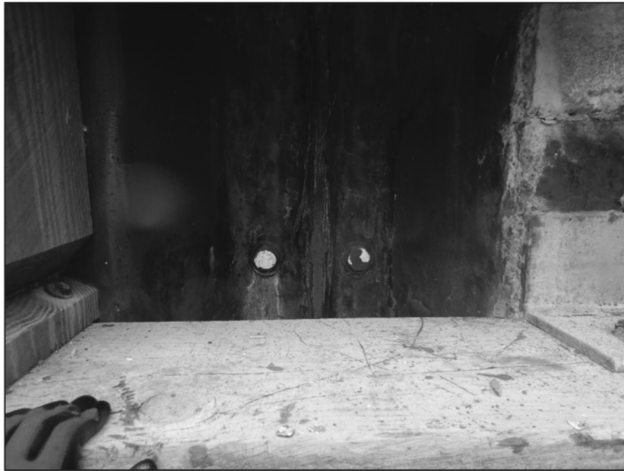
Photo 2-16 – Regular Washers on Tieback Assembly (Sta 70+00-97+50)
