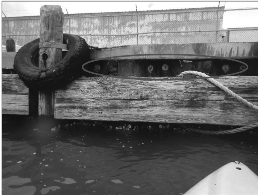
Photo 2-6 – Corrosion Holes at Top of Sheets (Sta 33+25)
