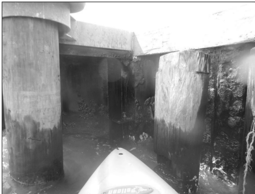
Photo 2-11 – Corrosion Hole at Transition (Sta 55+41), Concrete Fill Visible
