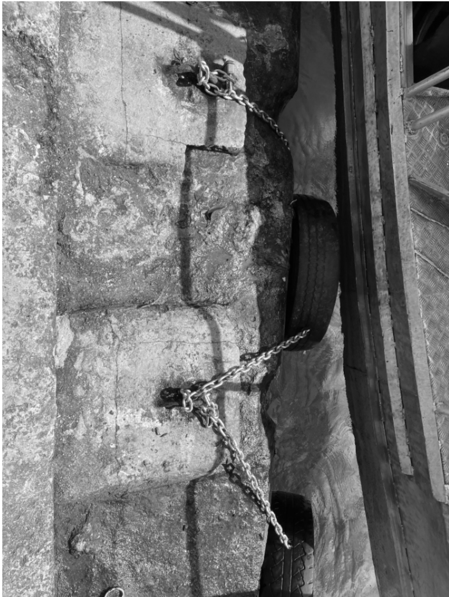
Photo 5 – Truck tires are used as fenders and hoisted using chains locked onto metal spikes drilled into the wharf. These are not made to handle vessel docking. The photo also shows the gap between the boat and the dock. Without a ramp, the wharf is not ADA accessible.
