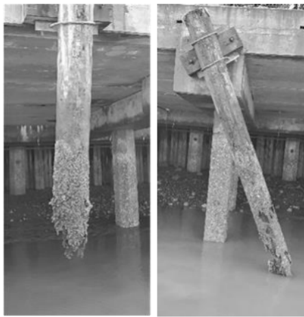
Figure 1. Examples of the failed and failing fender piles on the Fisherman's Terminal quay. All remaining pilings are in comparable condition, with five missing entirely.
