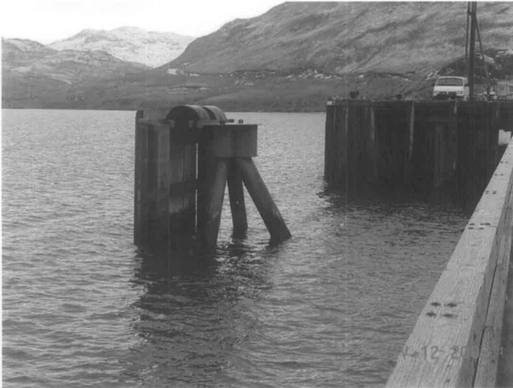
View of the North Dolphin and fender as seen from the north catwalk. The North Dolphin is in good condition.
