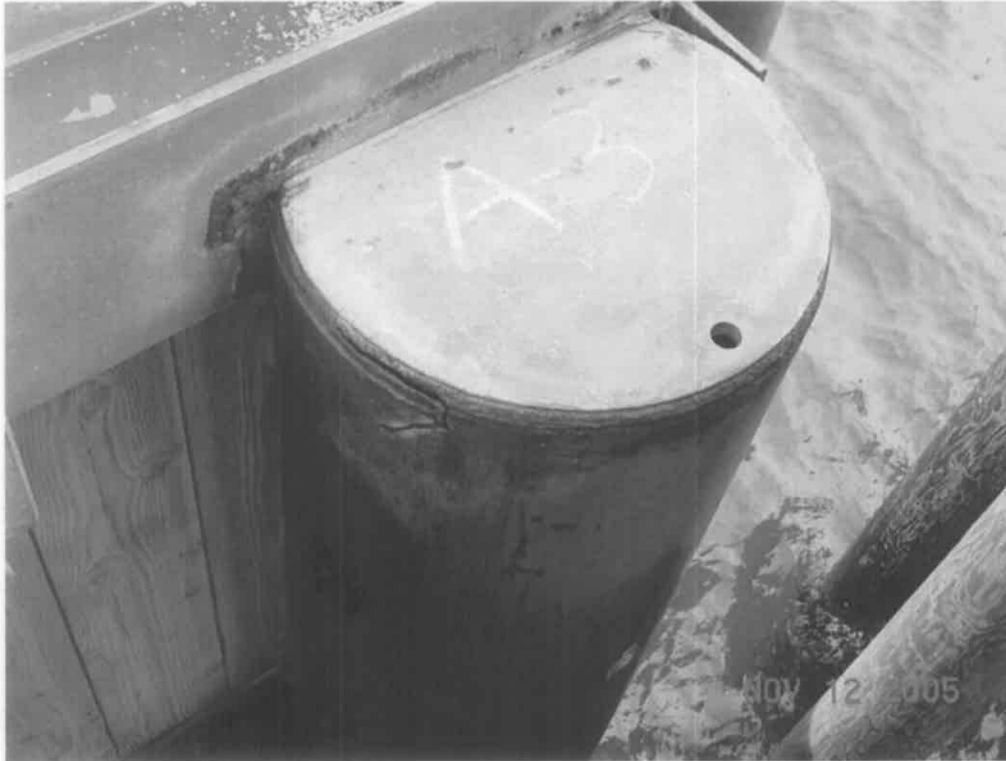
View of the broken and heavily corroded F3 fender pipe pile sleeve. This unit should be repaired and re-coated.
