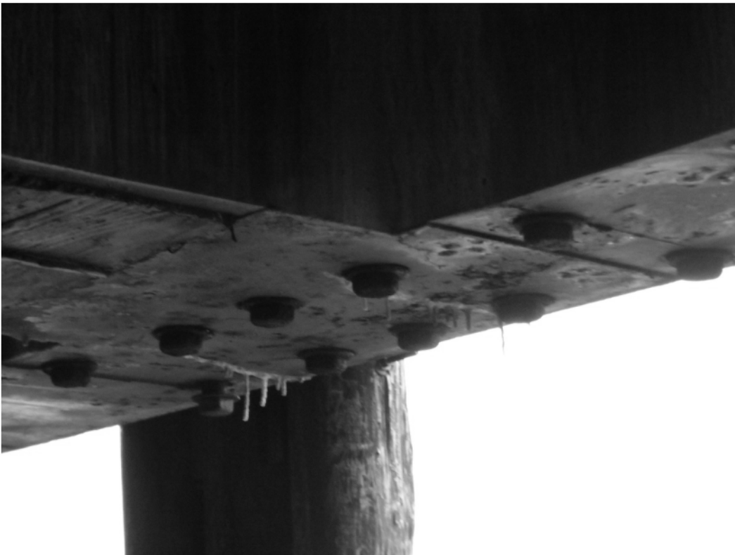
Photo P5-20. Bollard through-bolt connection under the pier, note the loose bolt.
