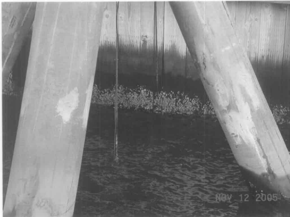
The pair of cables to the left supports and provides continuity to the anode that protects the dolphin piles and cap. The cables to the left act similarly for the fender framing steel. However, the brown support cable is broken leaving the anode hanging from only the black electrical continuity cable.
