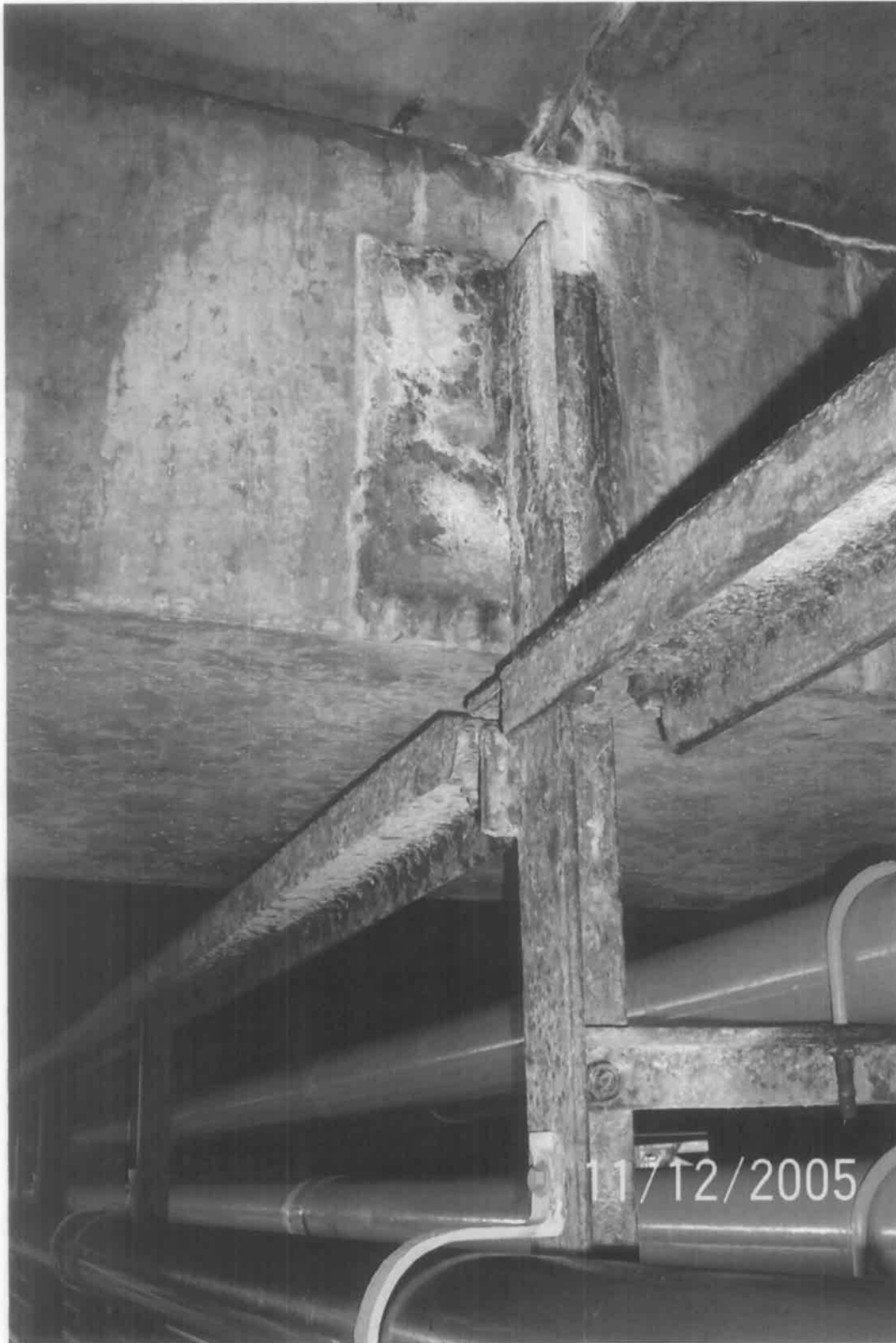
View of a similar connection in another location exhibiting very severe corrosion. This level of corrosion is common too much of the infrastructure beneath the dock.
