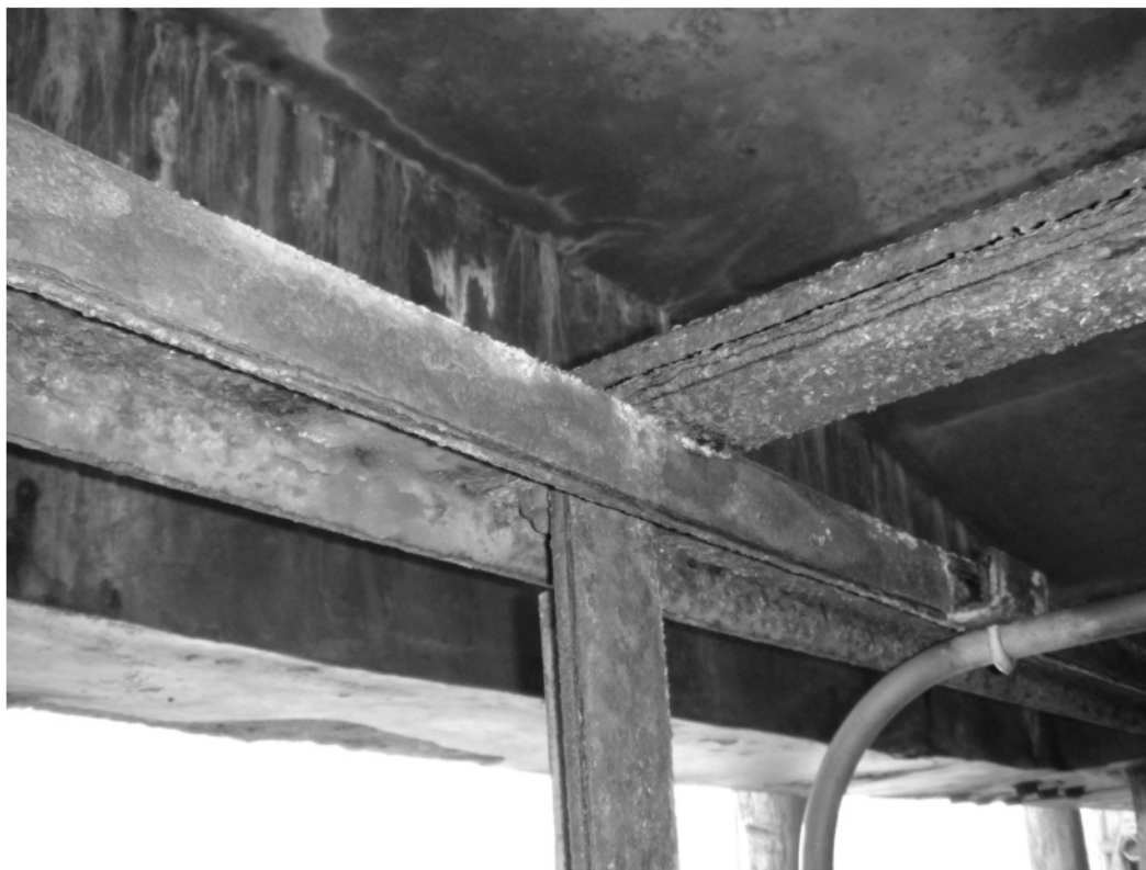
Photo P5-13. Severely corroded catwalk support members.
