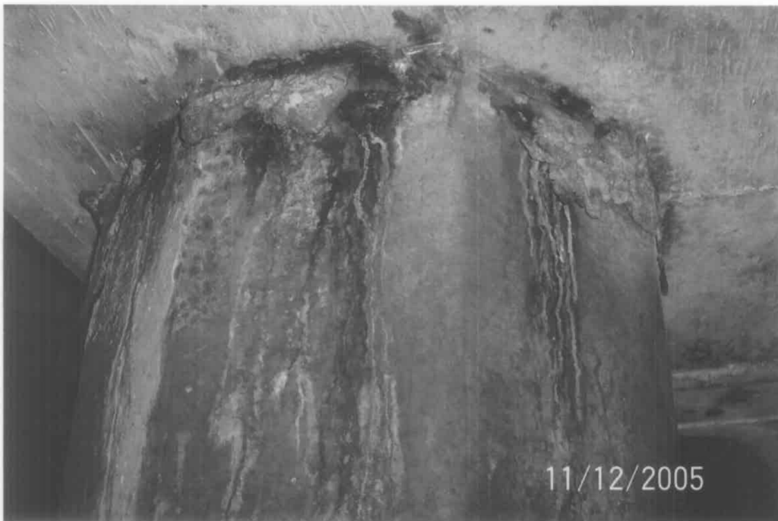
This pile-to-cap joint exhibits severe leaching of corrosion from the steel reinforcing inside the concrete. Water is entering the concrete, likely from above, and impacting the steel.
