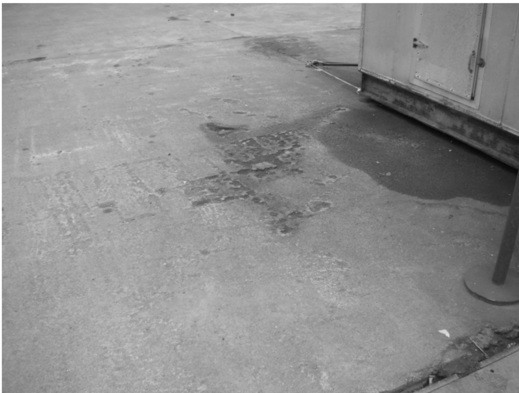
Photo P5-4. Area of localized damage on concrete deck topping slab.
