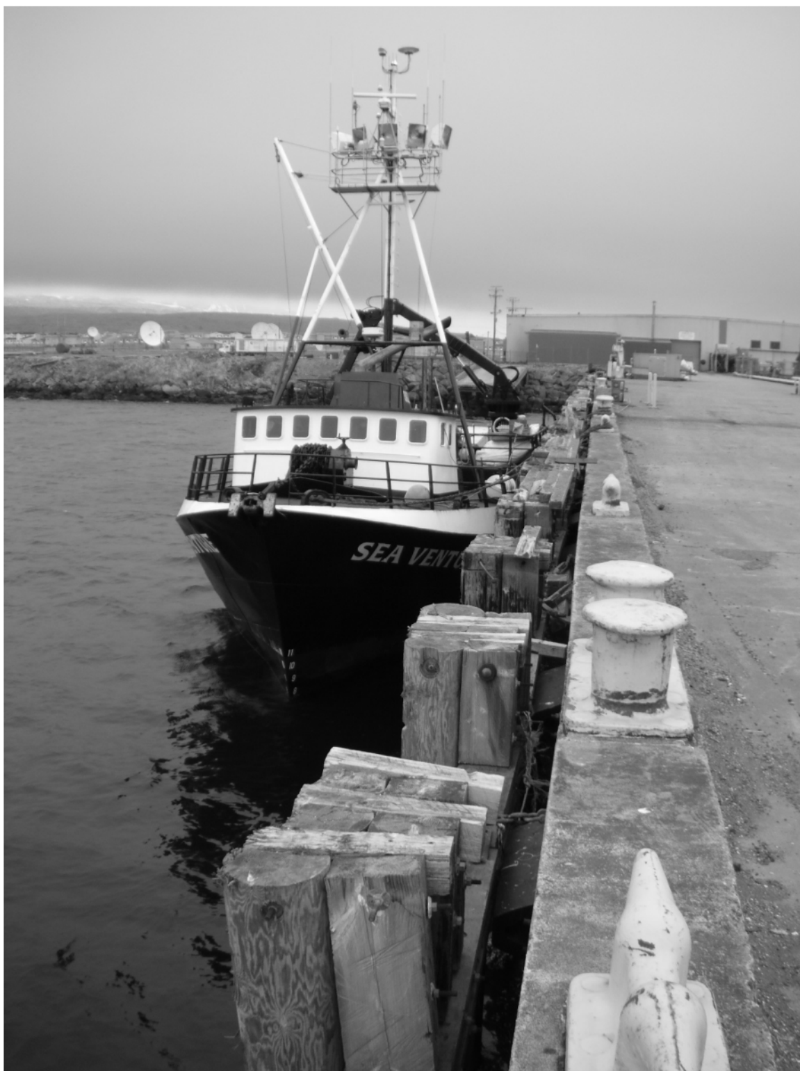
Photo P5-8. Dilapidated fender/waler system on west side of pier.
