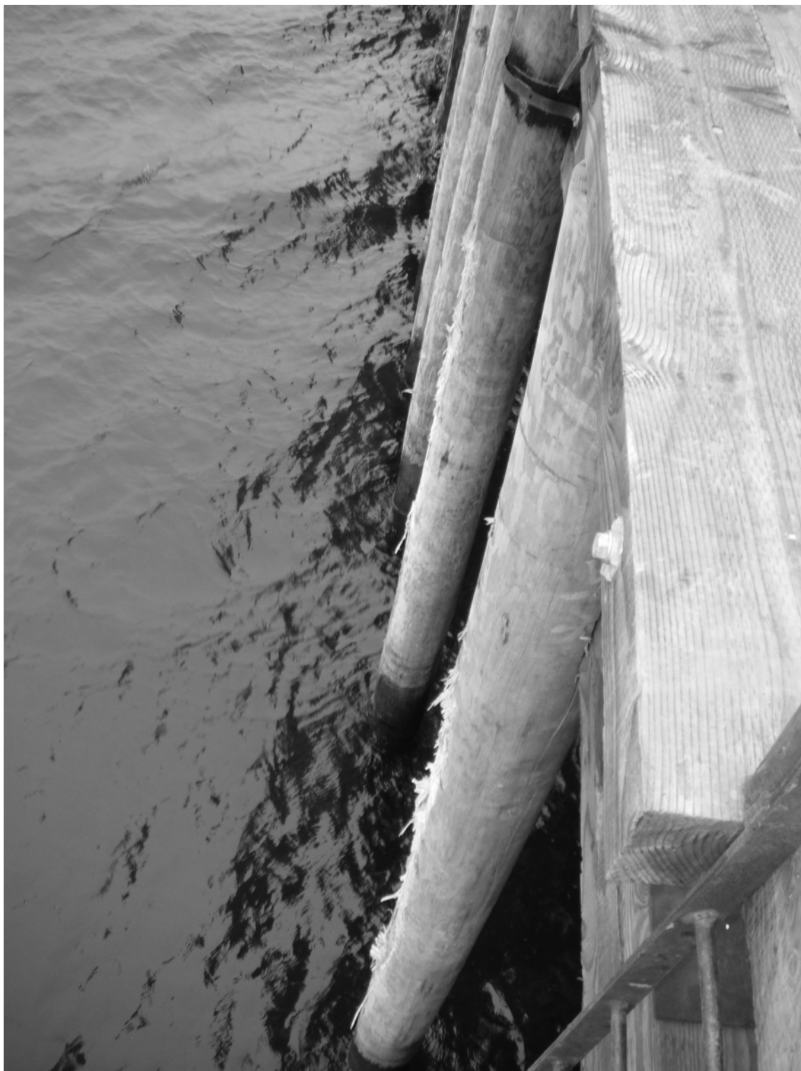
Photo P5-11. Abrasion damage on fender piles of replaced fender/waler section.
