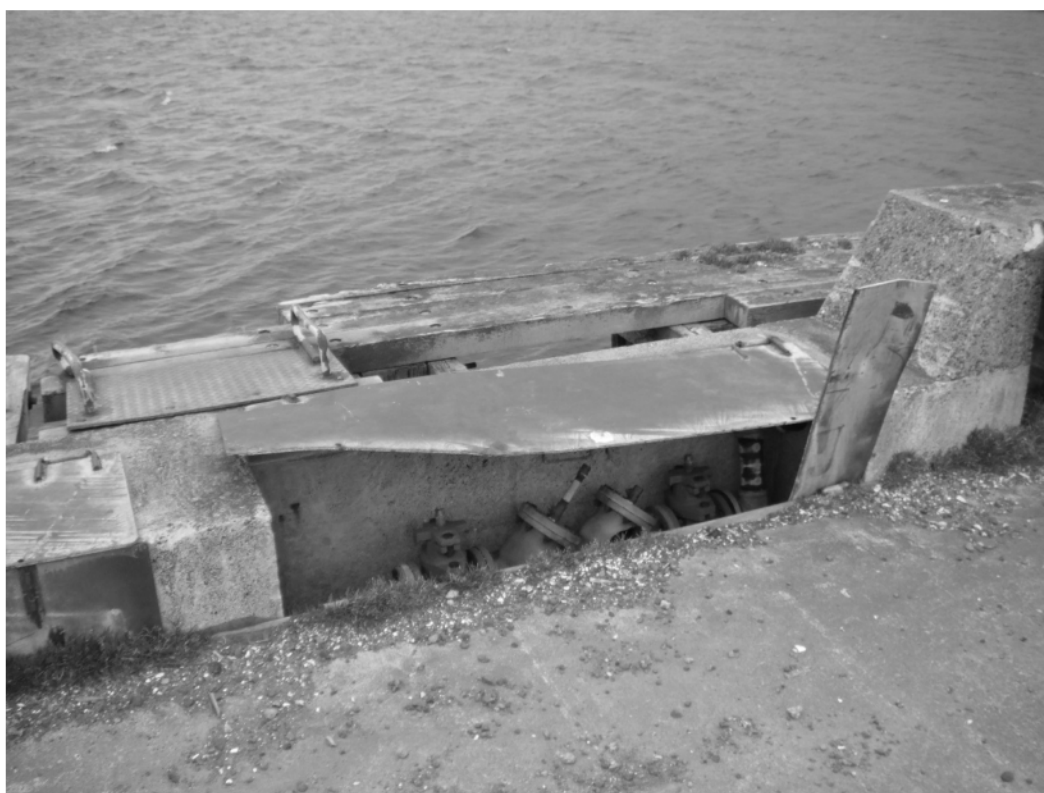
Photo P5-6. Damaged/missing covers for utility-way blockouts in bullrail.
