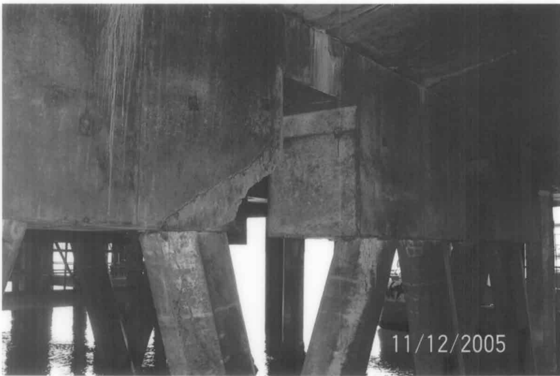
View of a large concrete spill on a cast concrete pile cap. Except for this damage and some minor leaching of water through the deck, the concrete on Pier #5 is in good condition.
