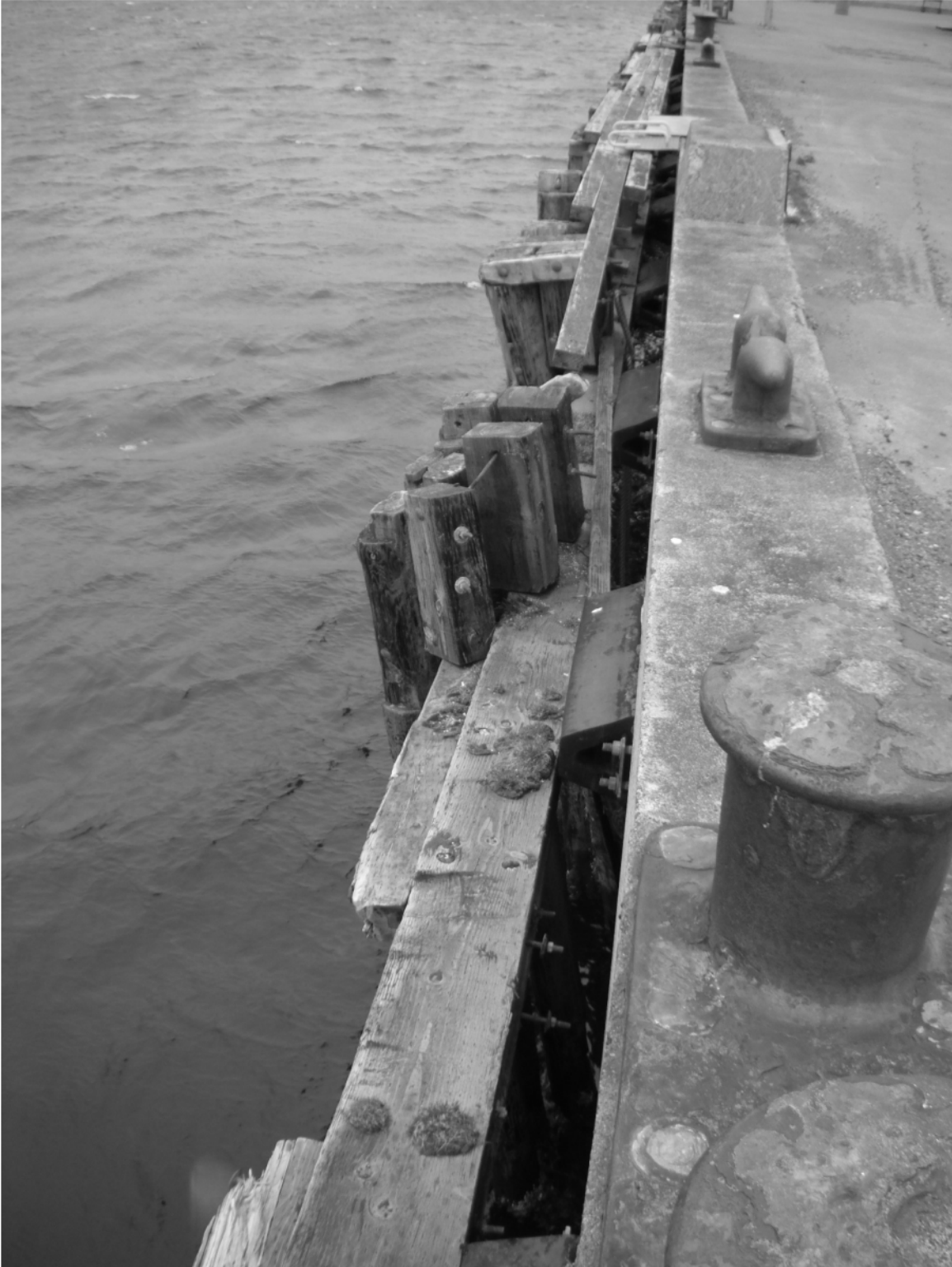
Photo P5-7. Dilapidated fender/waler system on east side of the pier.
