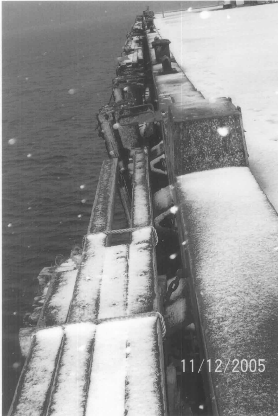
View sighting down the east side of Pier #5. The trapezoidal shaped energy absorbers can be seen behind heavily dilapidated fender/waler system.
