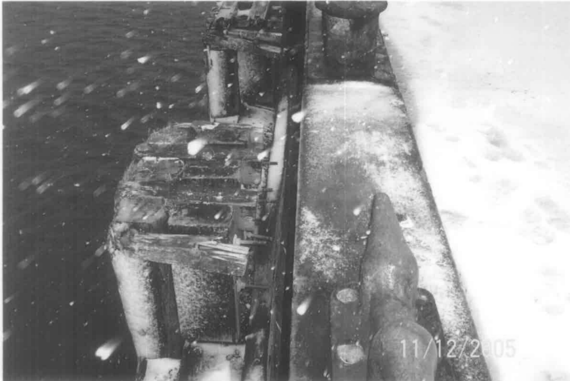
View of typical Pier #5 fender pile waler system at top of dock. The system is in very poor condition.
