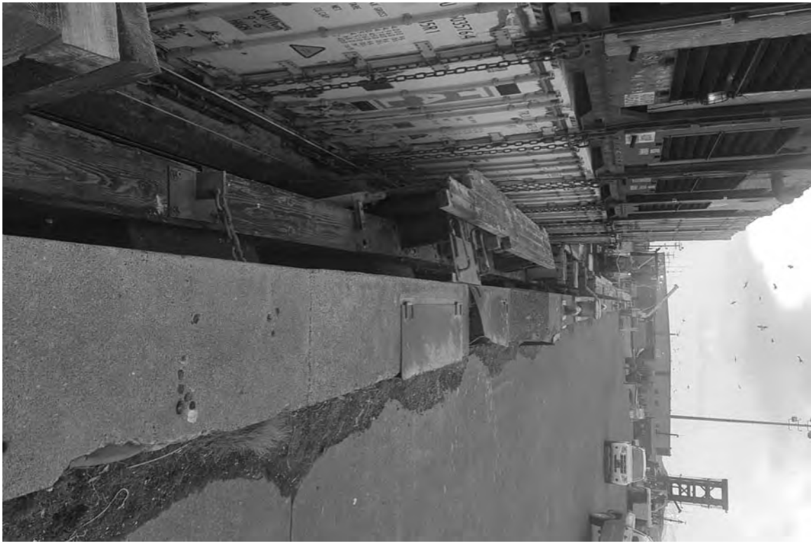
Barge alongside dock showing how compromised fender piles (angled) and proximity of barge life lines
