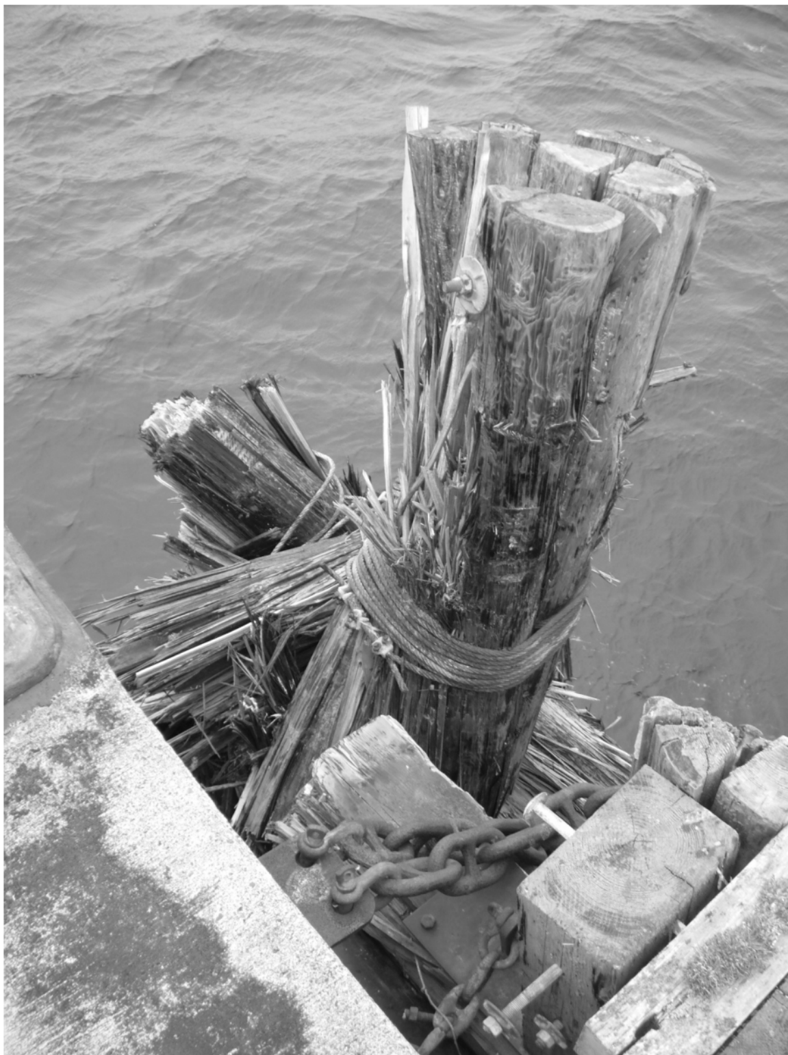
Photo P5-9. Severely damaged fender pile cluster at southwest corner of pier.
