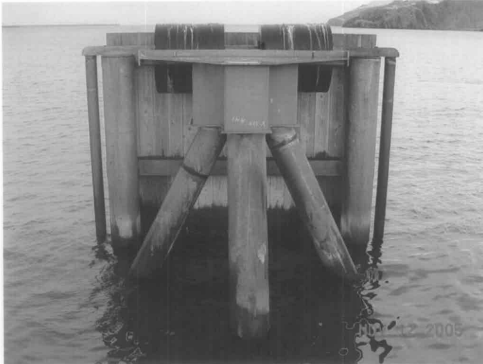
View of the South Dolphin and fender. Except for some minor corrosion and broken anode support cable it is in good condition.
