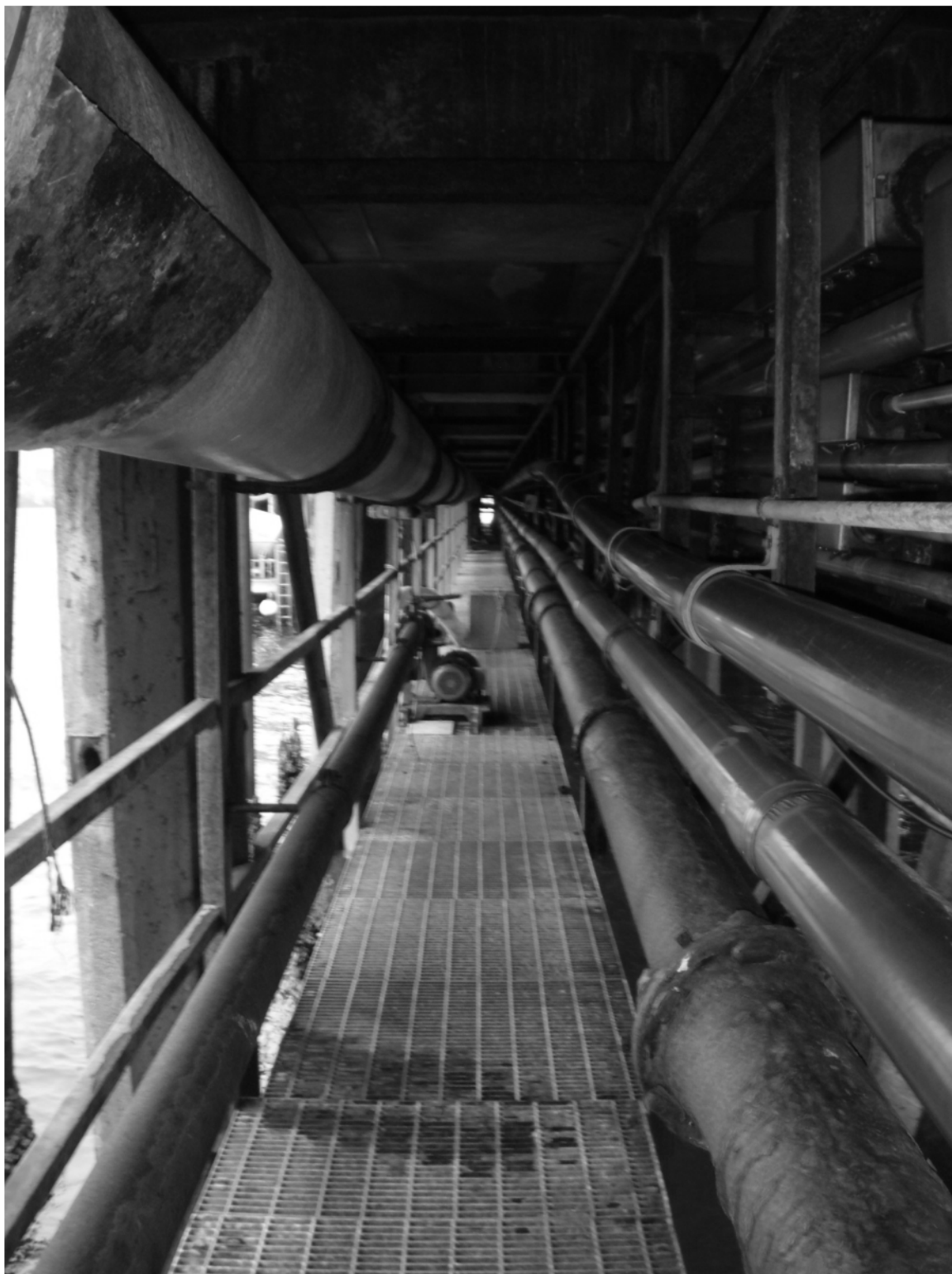
Photo P5-12. Catwalk and utilities under pier.
