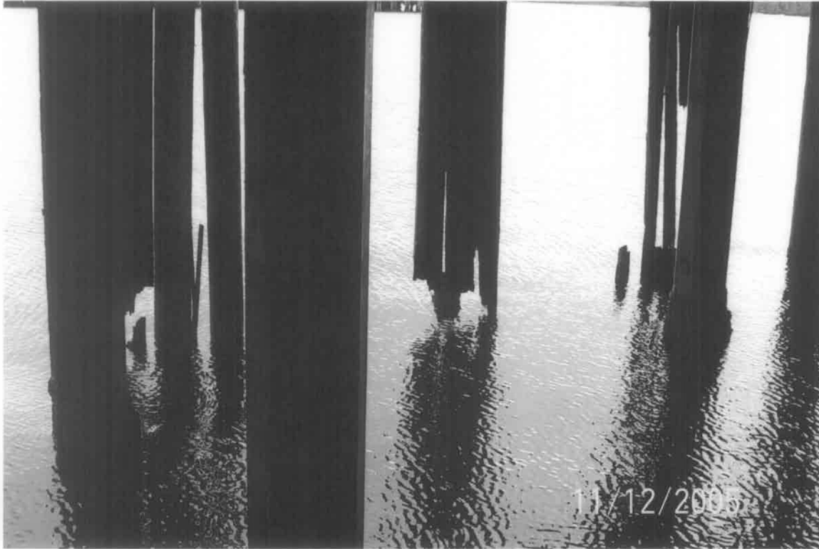
View of broken timber fender piles as viewed from beneath the dock.
