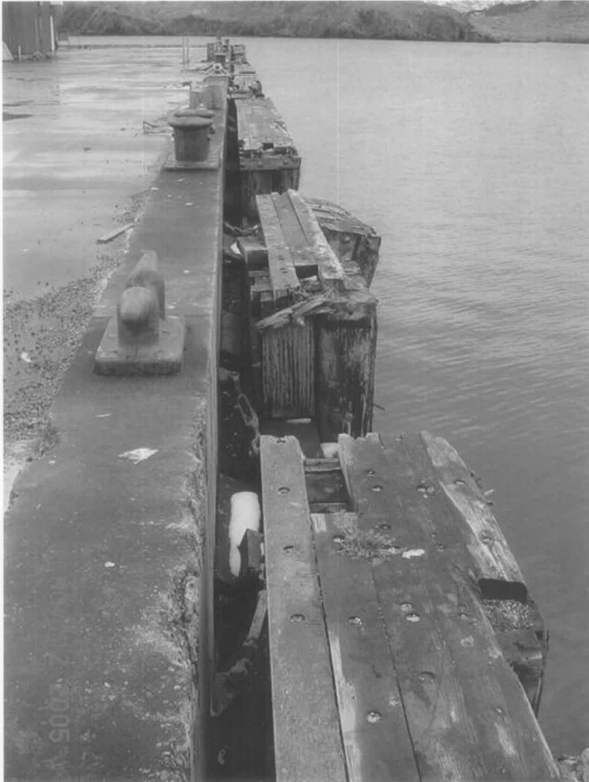
View sighting down the west side Pier #5. The entire top-side fender/waler system exhibited the broken and decayed timbers which are evident in this picture.
