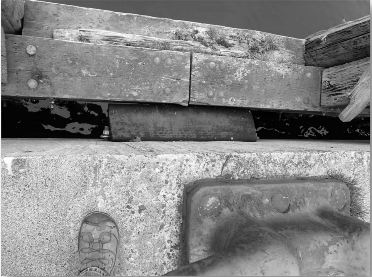
D rubber energy unit on the west face of Pier 5. (12 inches high, 8 inches wide, 3.5 feet long.)
