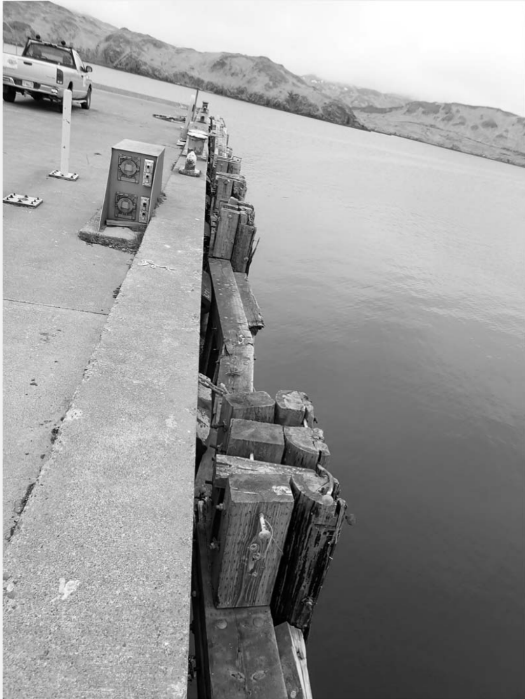
West face of Pier 5 2018 allision / damage area.
