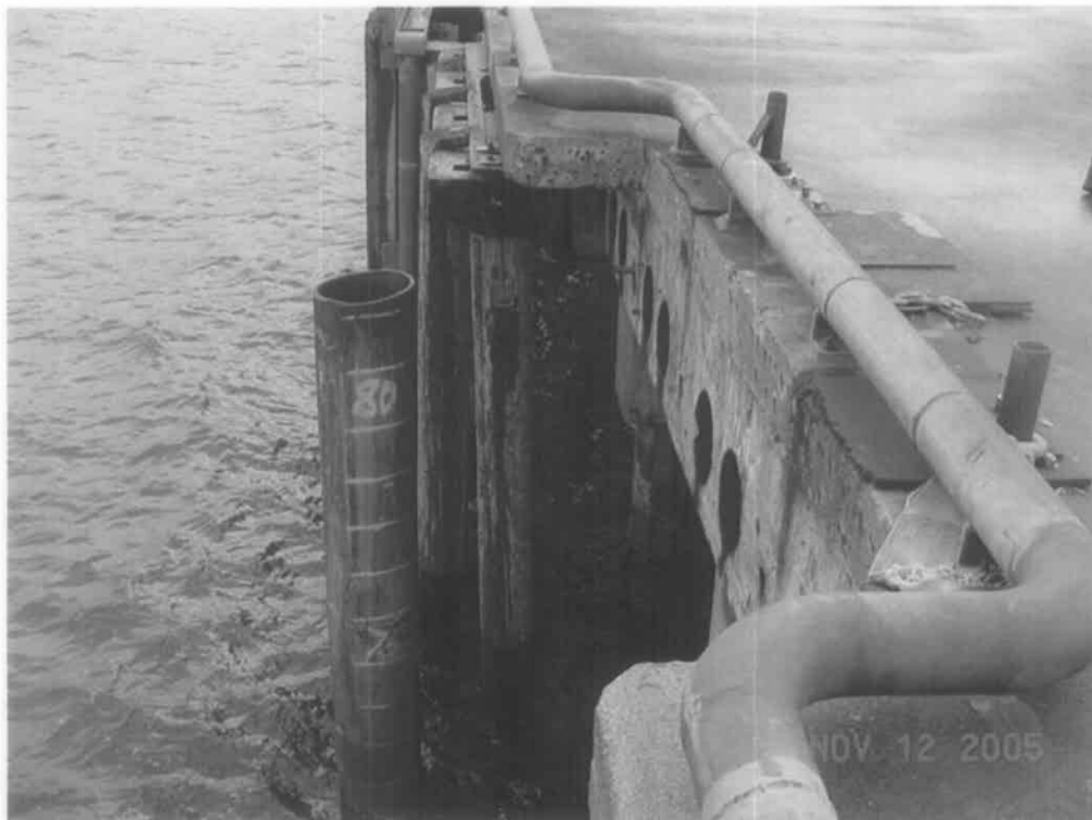
View of the missing fender unit at fender location F5. The visible pile is a pin pile which the fender pipe sleeves fit over. The other pin pile was missing. The fender should be replaced in the future.
