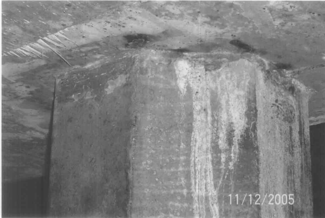
View of pile-to-cap joint where the concrete piling was cast into the concrete pile cap. This joint is in acceptable condition and did exhibit evidence of being re-grouted sometime after construction.
