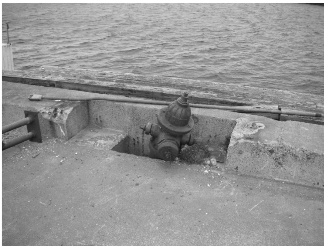
Photo P5-5. Damaged hydrant and detached line guard on west side of pier.
