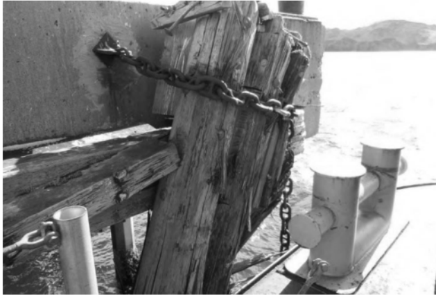
FIGURE 5 BARGE BOW DAMAGED FENDER PILE ASSEMBLY 1
