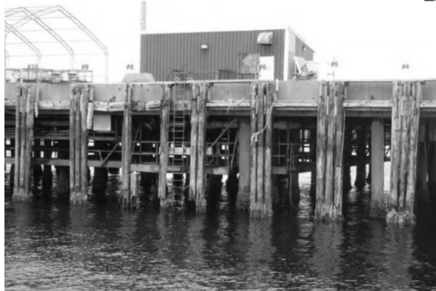
FIGURE 2 SAMPLE OF PILING DETERIORATION AT WATERLINE
