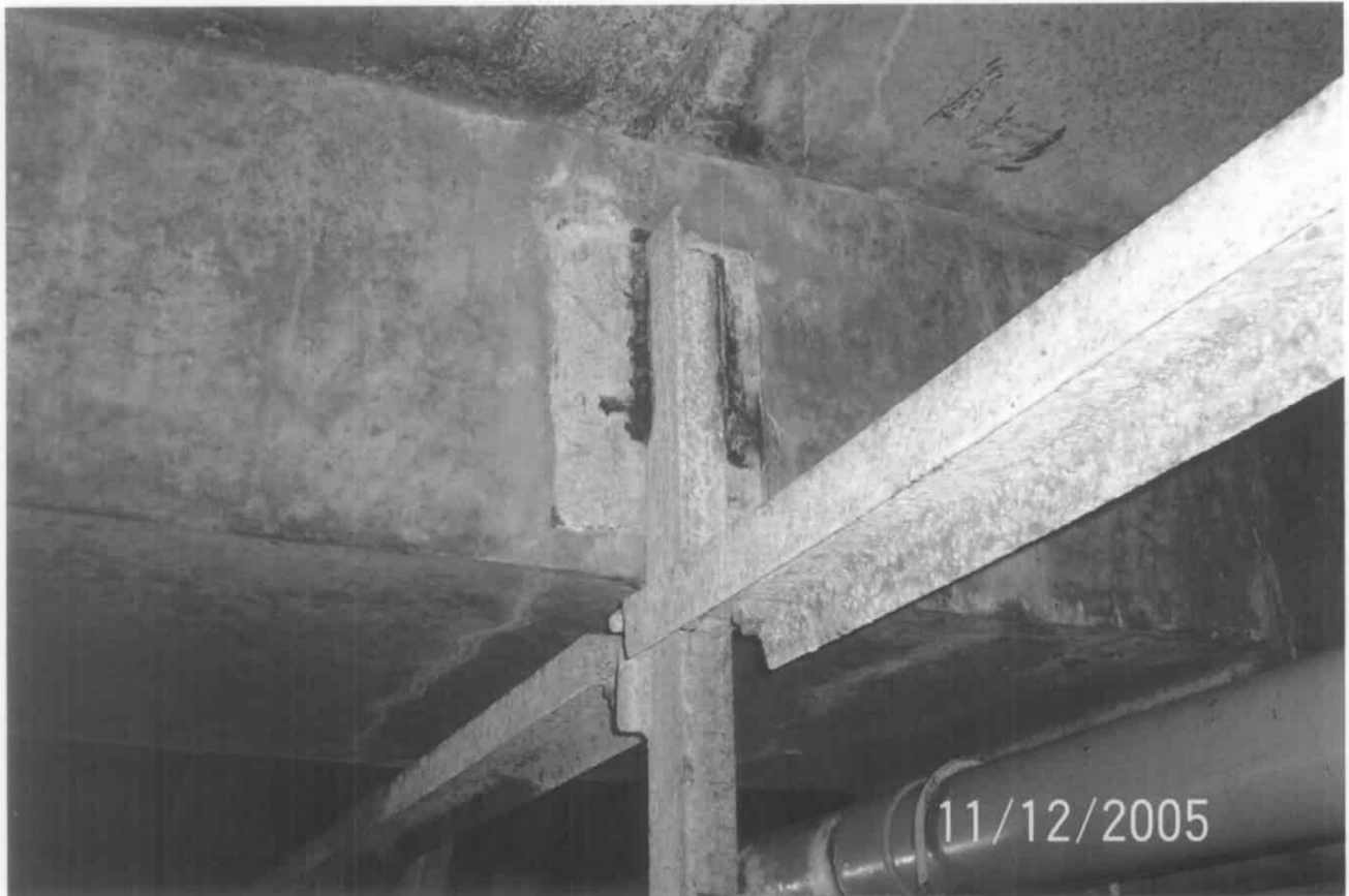
View of a plate cast into the concrete to provide an attachment point for utility hangers and brackets. This location was one of the points in better condition yet still exhibits corrosion and is in need of repair.
