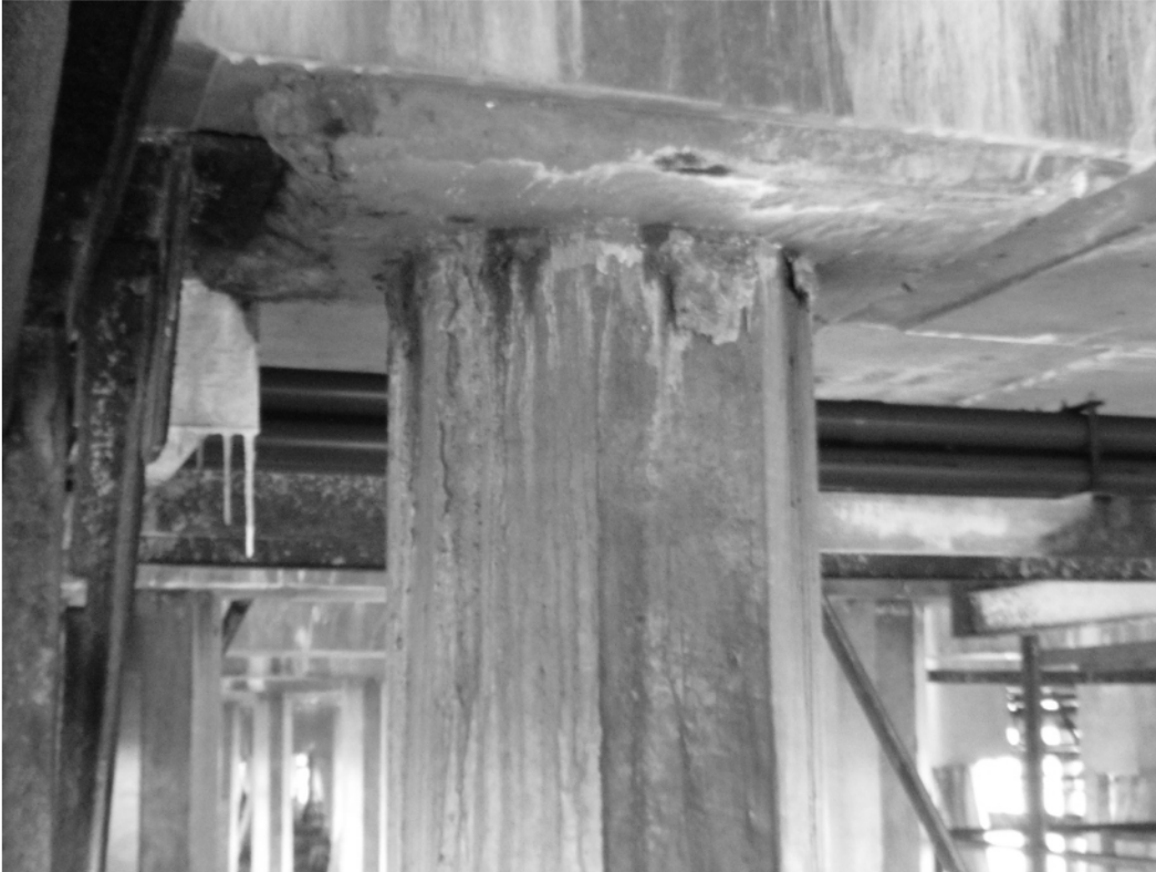
Photo P5-19. Corrosion staining at top of support pile from pile cap attachment.
