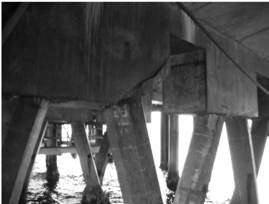
Photo P5-17. Spalled concrete pile cap at grid 11D.
