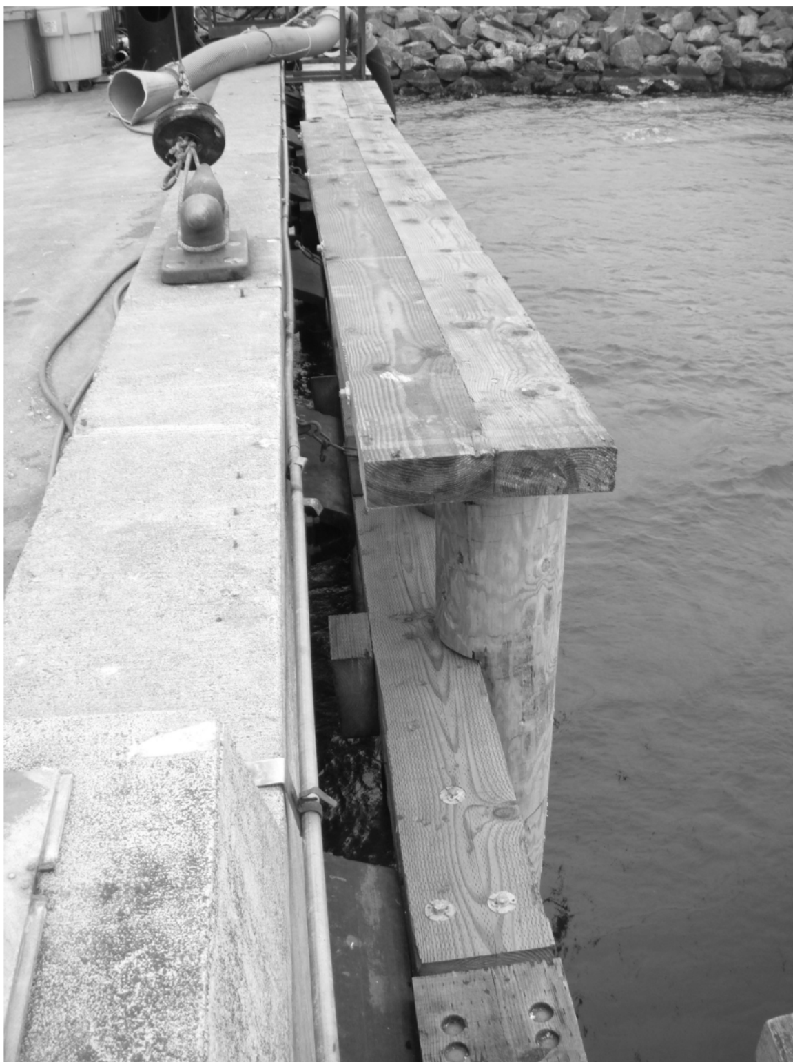
Photo P5-10. Replaced section of fender/waler system in front of crane at northwest corner of pier.
