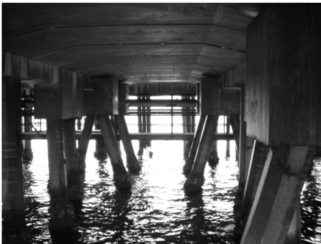
Photo P5-15. Deck panels, pile caps, and support piles under the pier.
