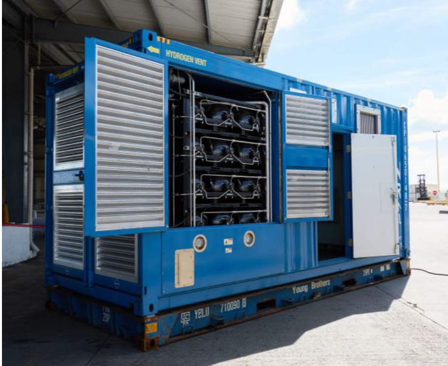
Figure 2. The 100-kW MarFC unit, with integrated hydrogen storage, PEM fuel cell and power conditioning equipment. The containerized MarFC is 19'10.5" long, 8.0' wide, 8'6" tall, and weighs approximately 25,000 lbs.
