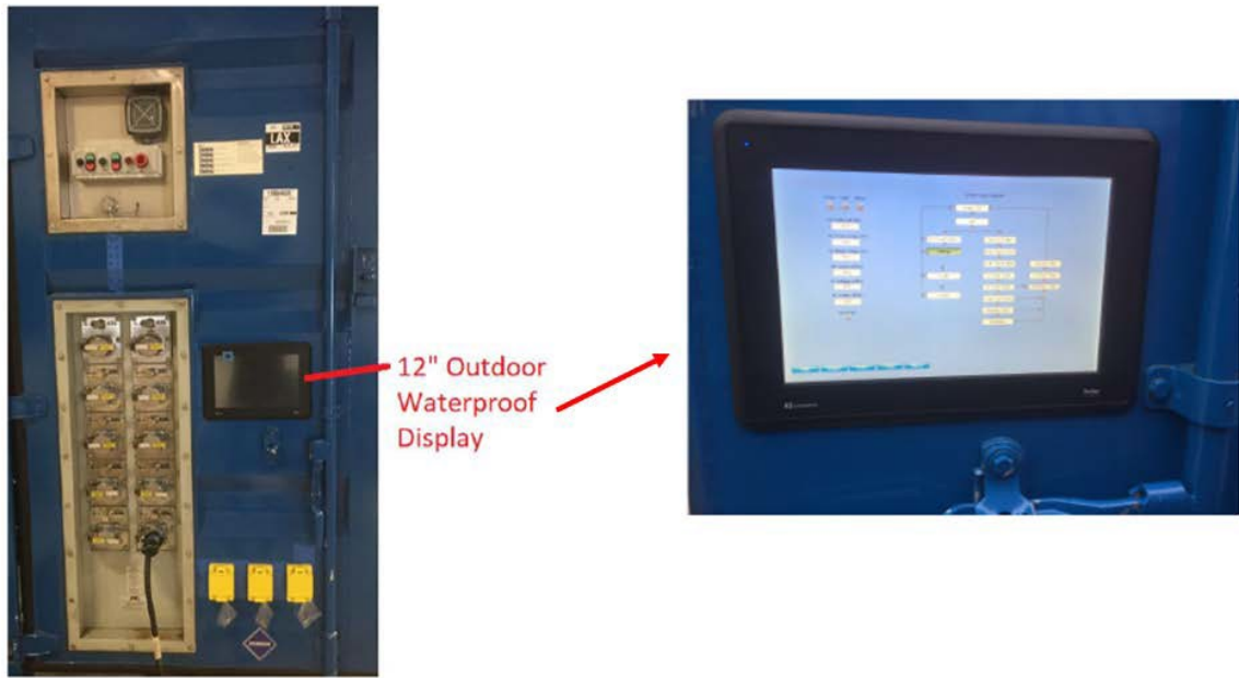
Figure 6. Installation of a ruggedized system display, making it easy for the operator to ascertain the state of the MarFC, especially during start-up.
