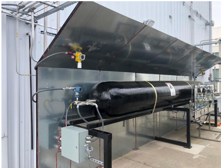
Figure 2: Example of the Type IV Composite Tank from Hexagon Purus planned for the Discover Zero. Photo Credit: Bikram Roy-Chaudhury, Air Liquide.
