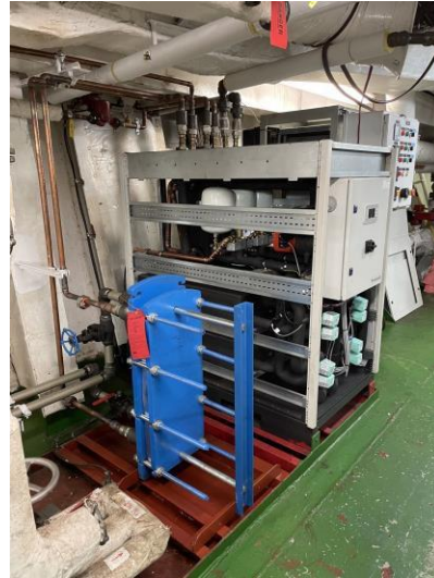
Figures 6 & 7 - Thermal Energy Conversion Equipment (Waste Heat Driven Adsorption Chiller) and Seawater Heat Exchanger installed
