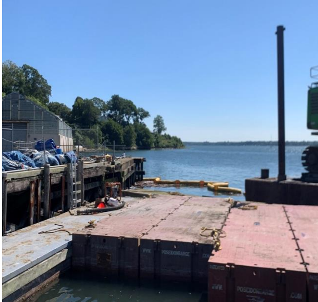
Demolition of Crowninshield Pier
