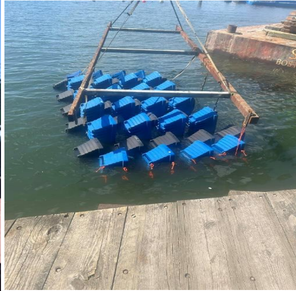
Installation of temporary wave attenuator
