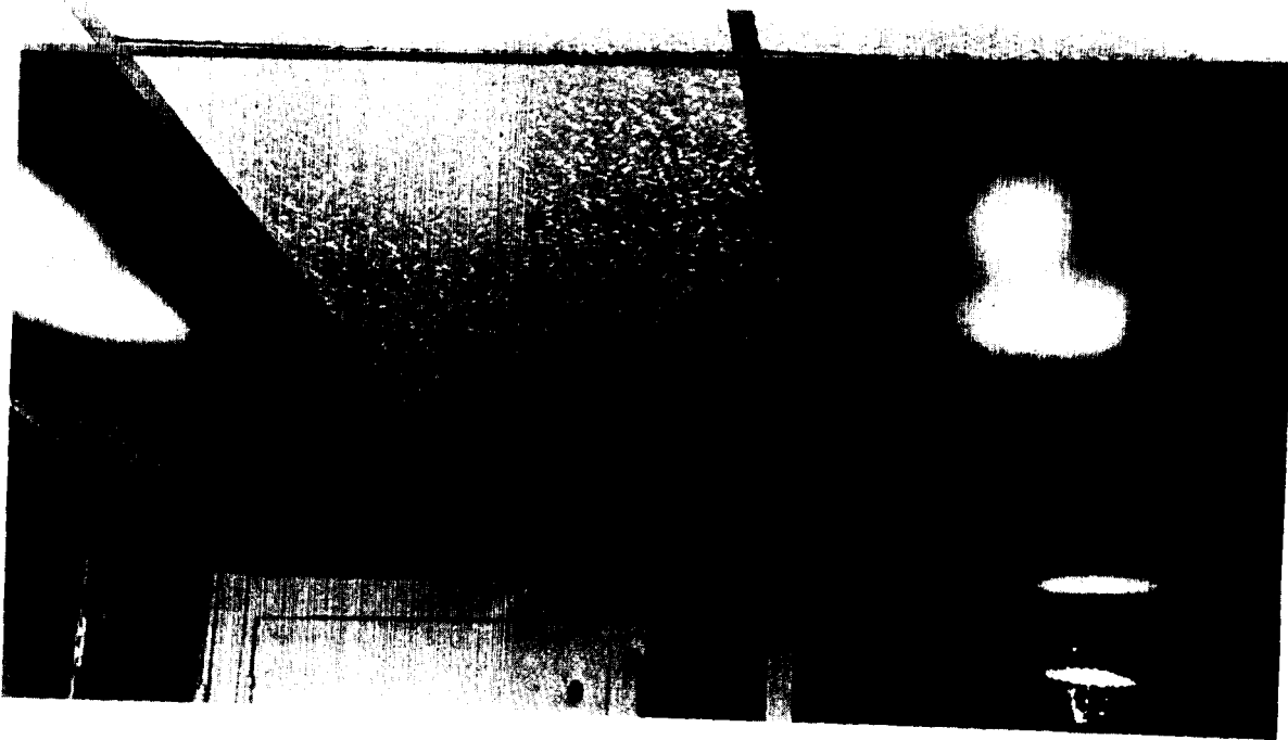
FIGURE 118. Spotty illumination results when improper lighting fixtures are used in type of overhead sheathing. (For proper installation see method E-7-A of appendix B)
