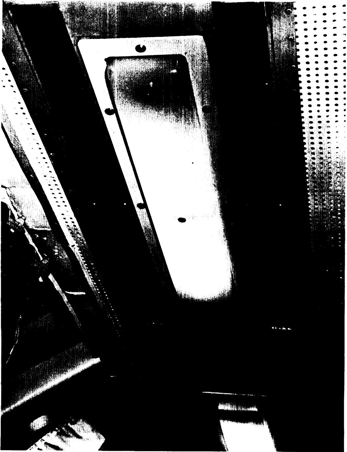
FIGURE 103. Typical flush mounting of fluorescent lighting fixtures. (For details see method E-1-B of appendix B)
