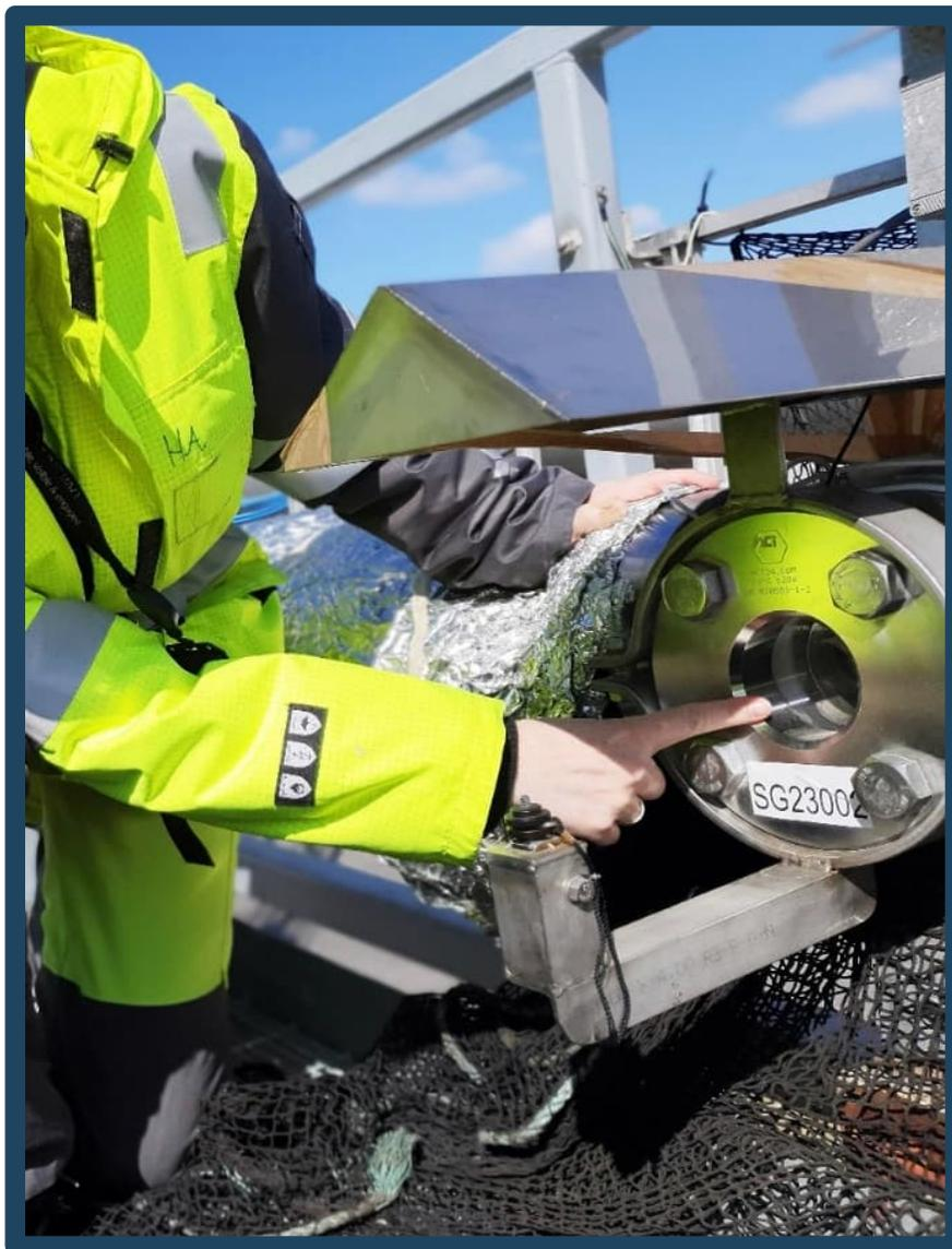
Figure 9. Inspection Window in LCO<sub>2</sub> pipeline (credit: Siri Krohn-Fagervoll)
