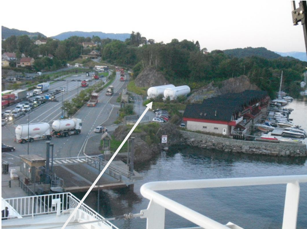
Photo 3: Dedicated 500 m 3 LNG storage tanks at ferry terminal in Halhjem, Norway
