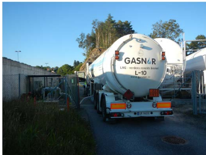
Photo 4: Resupply of LNG storage tanks from a road truck
