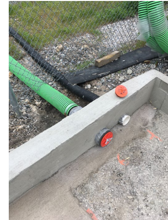
Secondary sump drain layout
