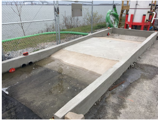
Dewatering pad overview
