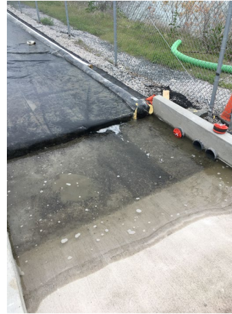
Drains in normal operation
