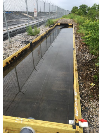
Post construction inflow side
