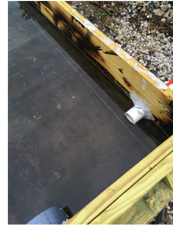
Inflow pipe and drain pipe
