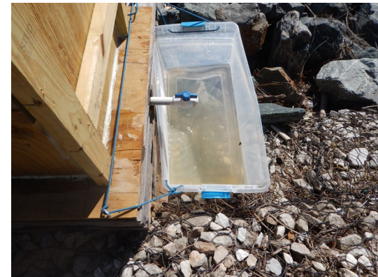
Draining with typical effluent
