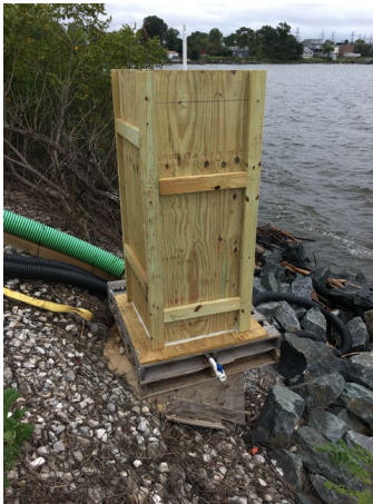
Final and in place
