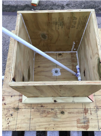
Drain and air break PVC
