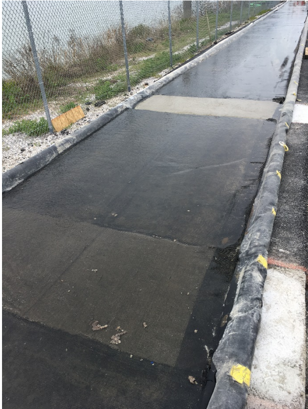
Figure 2-7 Two Algal Flow-way Sections with Roughened Concrete Surface
