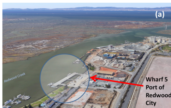
Figure 31: Location of Wharf 5, Port of Redwood City, Redwood City CA. (a) General Wharf 5 location relative to the San Francisco Bay; (b) close-up view of the Zero-V docked at Wharf 5 along with two LH 2 trailers and refueling stanchion show in red. The refueling stanchion is notional only. The relative sizes of the Zero-V, LH 2 trailers and dock are properly rendered. Satellite images are courtesy of Google Maps.
