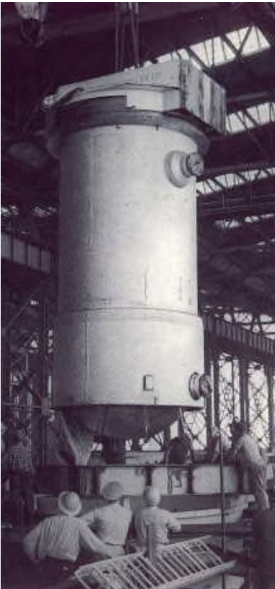
Figure 7-2 Reactor Vessel during Fabrication
